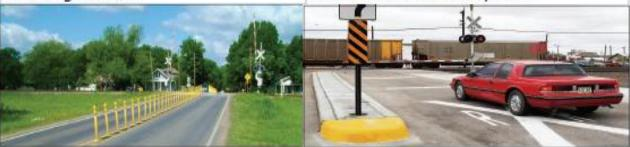
Gates with Channelization Devices Gates with Medians
