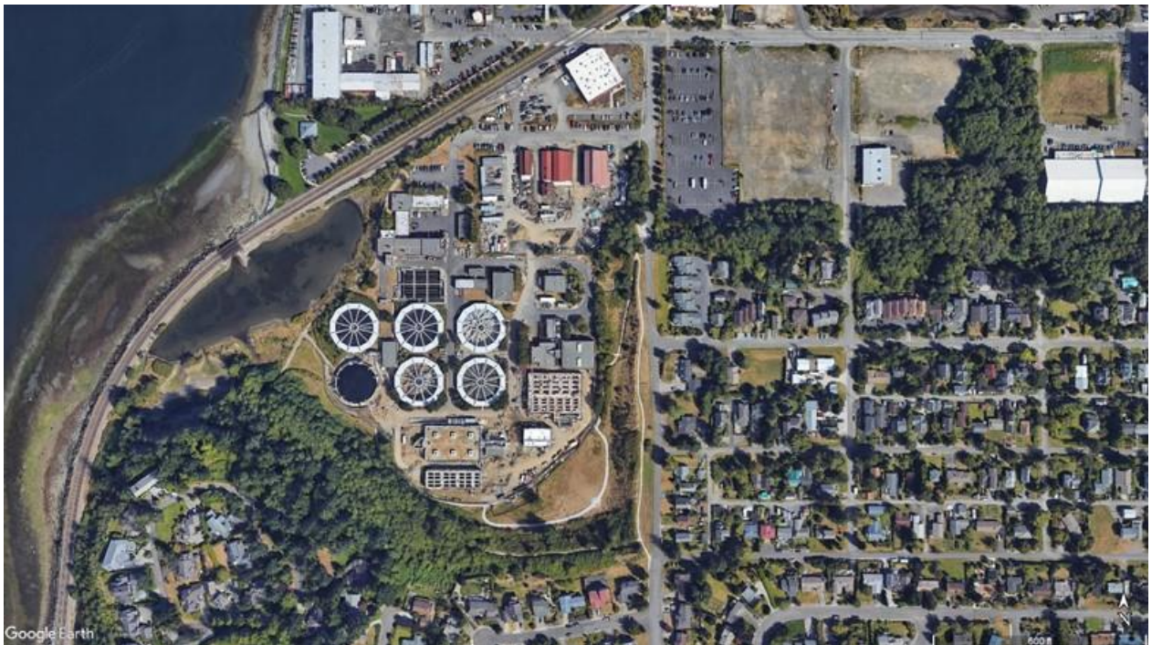
Figure 1. Aerial view of the Post Point Wastewater Treatment Plant
