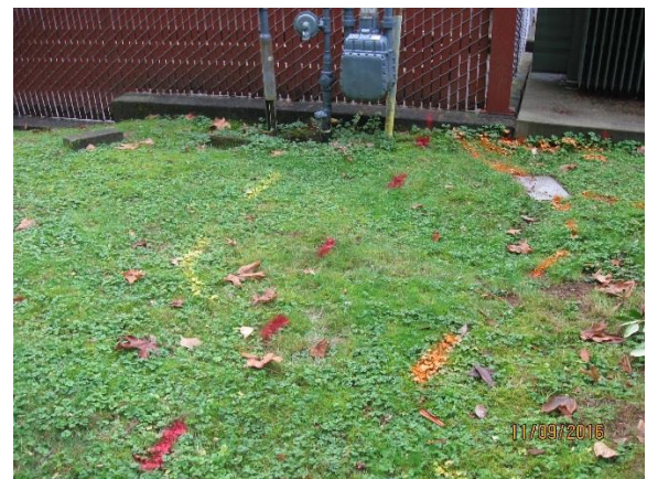
Starts with marking - or placing "locate marks" - where the utilities are, before disturbing the ground.
