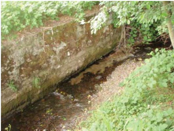
Note undercutting by erosion in some areas along the creek waterline. The base of the upstream retaining wall, view northeast. 2012
