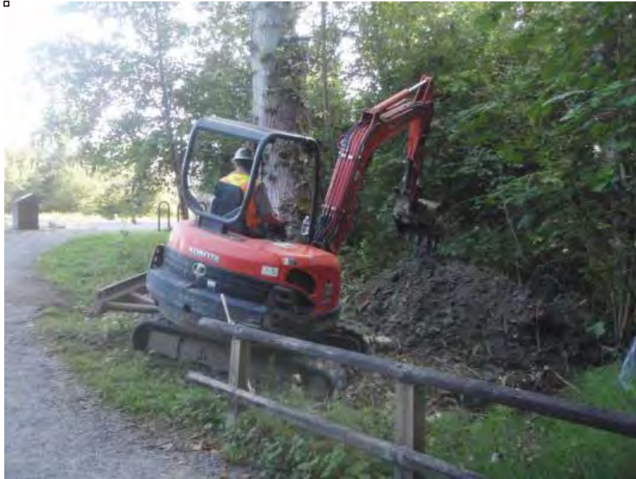
Figure 10. Backhoe excavating geotest trenches along the APE within the park.
