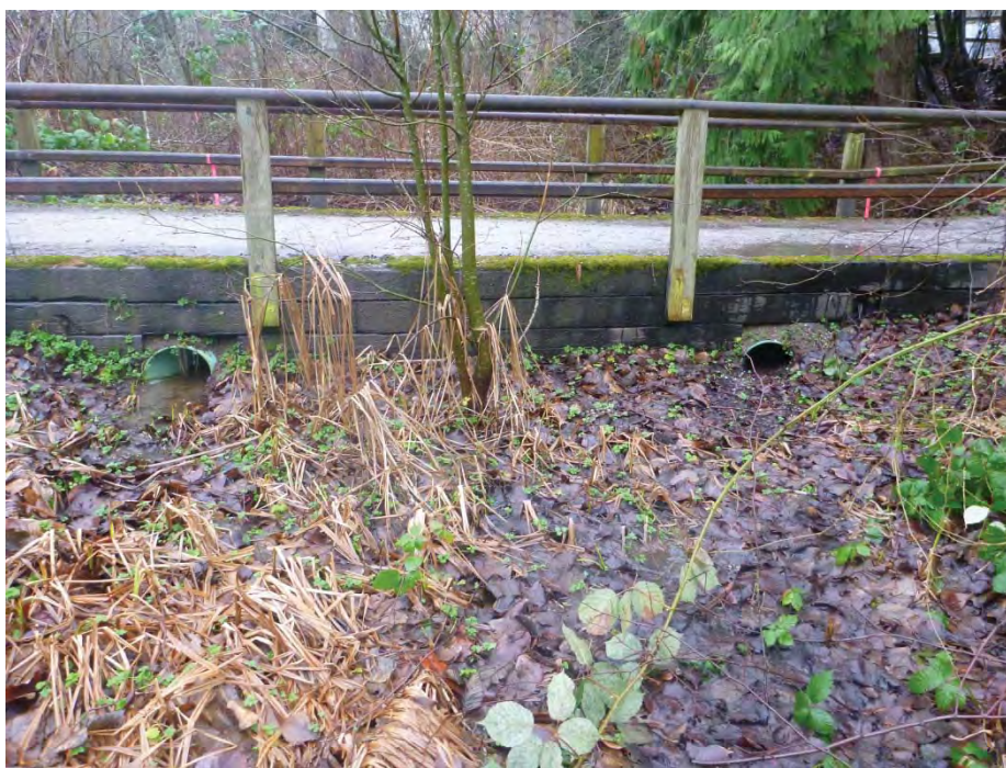
Photograph 5 Two culverts beneath walking trail that appear to have intermittent surface water connections between Wetlands A and B
