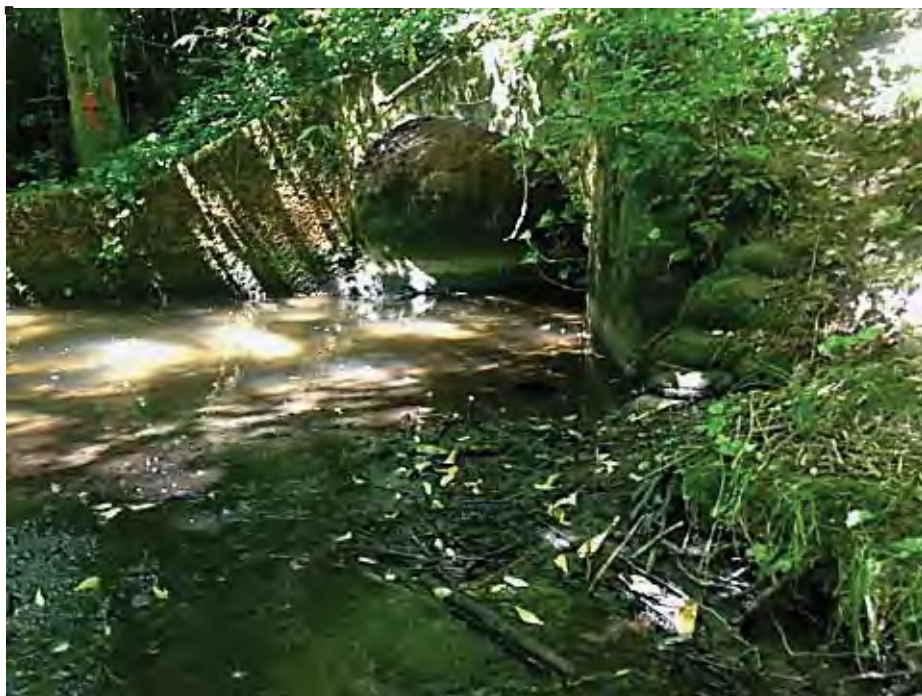
Figure 19. The downstream headwall, view northeast (courtesy of Aaron Hartvigsen, GeoEngineers Inc.). Note the retaining wall reinforcement along the southeast wing wall.
