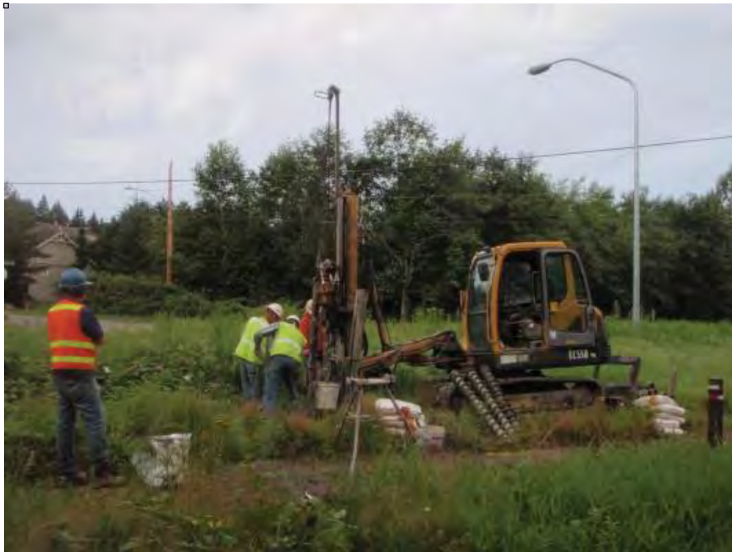
Figure 8. Auger excavating geotest borings along the eastern APE.
