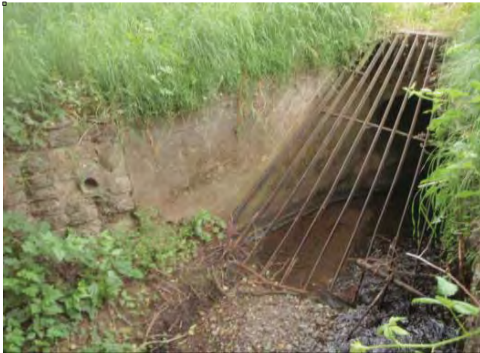
Figure 15. The upstream headwall, view southwest. Note the retaining wall reinforcement along the south wing wall.
