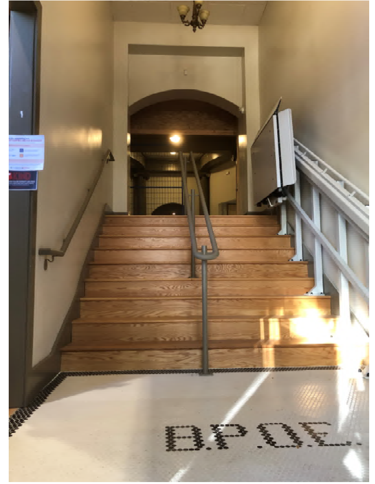
Platform Lift at Sidewalk Entrance Level
