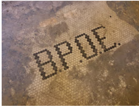
Original Mosaic under Tile – January 2020
