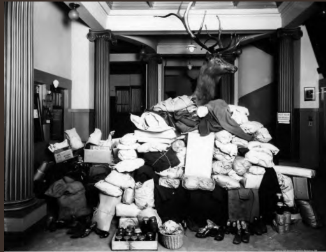
First Floor Entry Lobby, 1925 – Courtesy of Whatcom Museum
