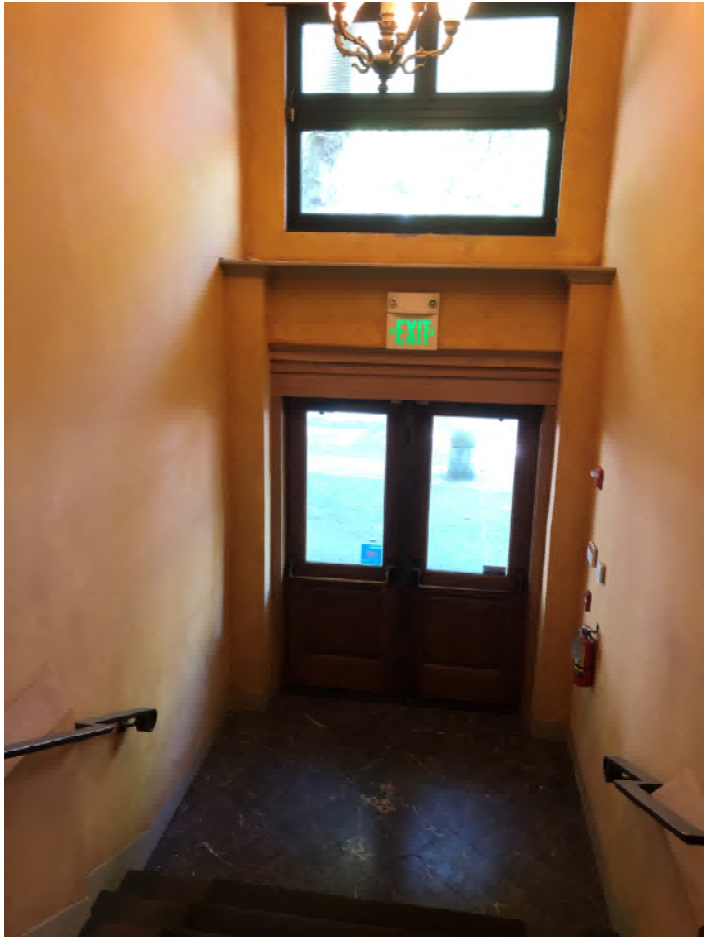
Existing Entry Lobby Tile – June 2019
