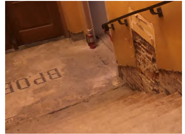
Original Mosaic under Tile – January 2020
