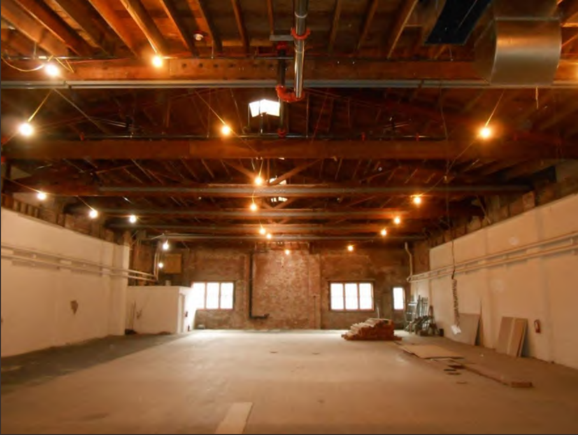
Second Floor Former Lodge Space, 2018
