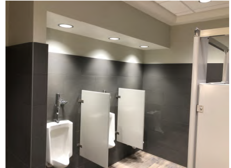
Typical Stall Finishes
