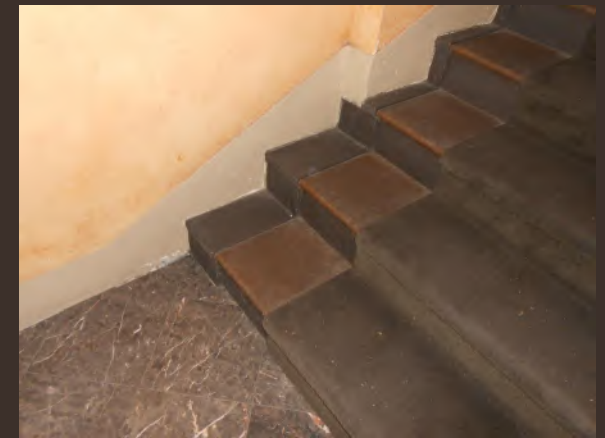
First Floor Entry Stair Detail, 2018
