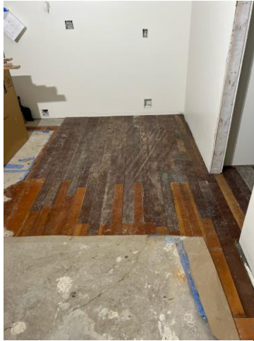
Patch over old bathroom
