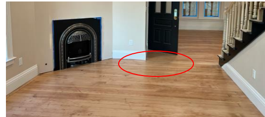
Refinished existing wood. Patches at removed wall.
