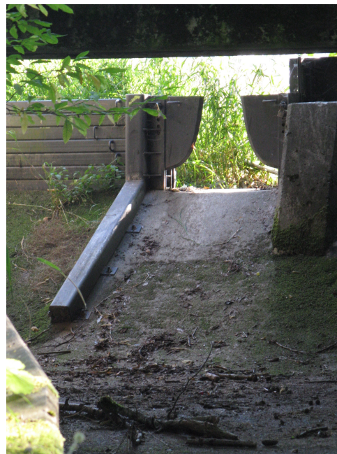
Figure 7.0-2. Dry control gate spillway at Lake Padden in September of 2011.
