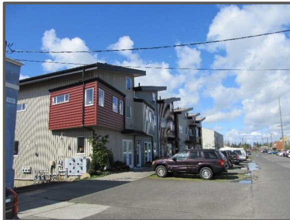
Live/work units on Ellis Street.
