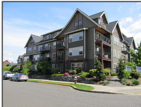
Multi-family units on High Street.
