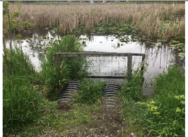
Beaver cages on west ends of pipes under public trail in center of Scudder Pond (4/30/2018)
