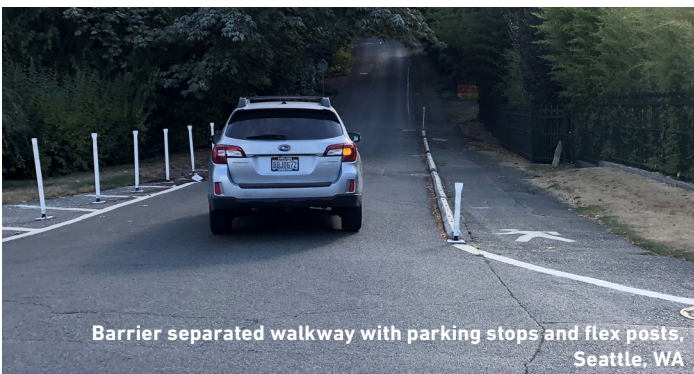
Alternative Walkway with wheel stops, Seattle, WA
