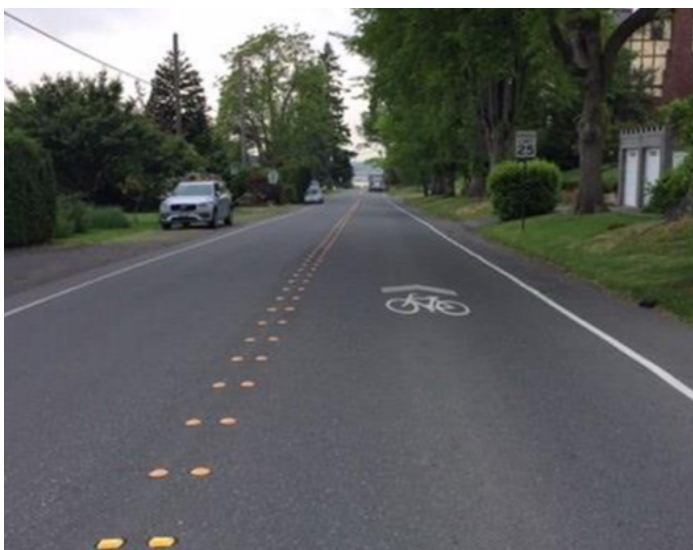
Arterial shared lane markings on 14th St in the South Hill Neighborhood
