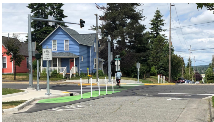
Bike HAWK crossing on Lakeway Dr on the Grant Street Bike Boulevard, including green crossing markings, short sections of green receiving bike lanes, a refuge island, and a diverter
