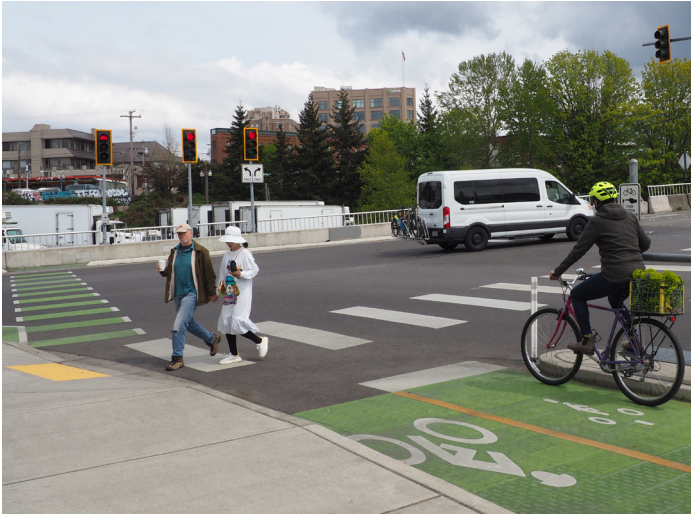
Dedicated Bicycle Signal on Granary Ave at Roeder Ave with Push Button Actuation and a Bicycle Stand
