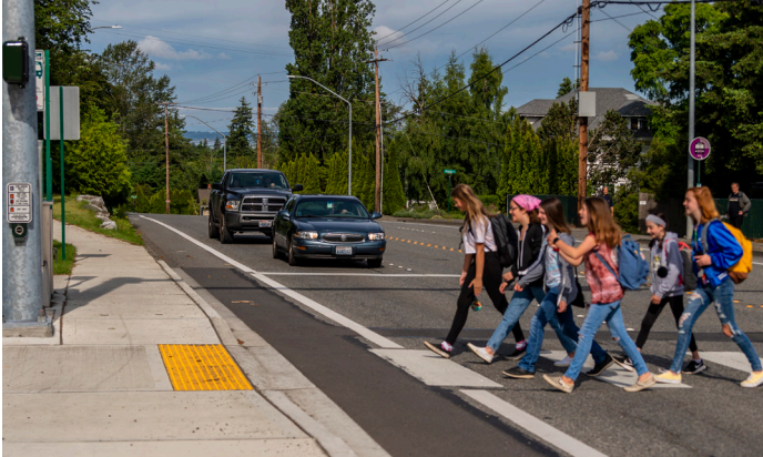
Crosswalk, curb ramp, and advanced stop line in Pedestrian Hybrid (HAWK) Signal on Lakeway Dr at Undine St
