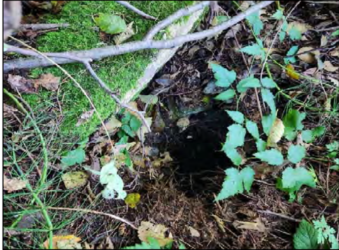
Photo 16: Found SD inlet at East edge of LHA basin and site, leads to Sea Pines Road utility. (10-7-24)
