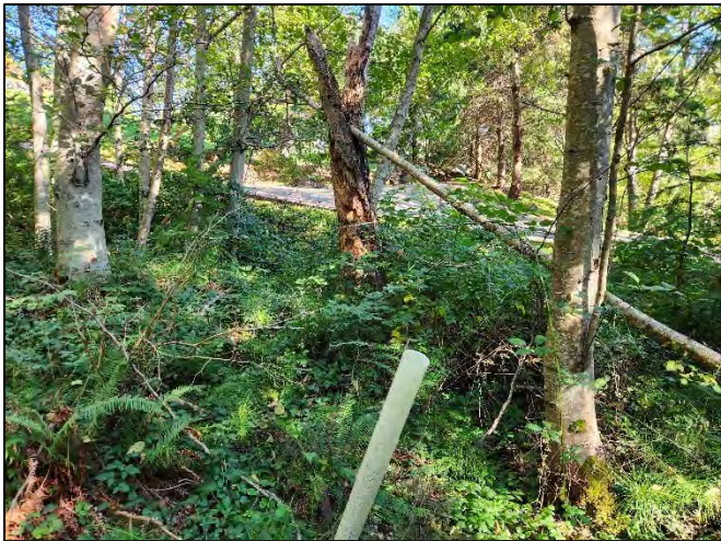
Photo 15: Within east side of LHA basin, looking east toward SFR driveway embankment. (10-7-24)
