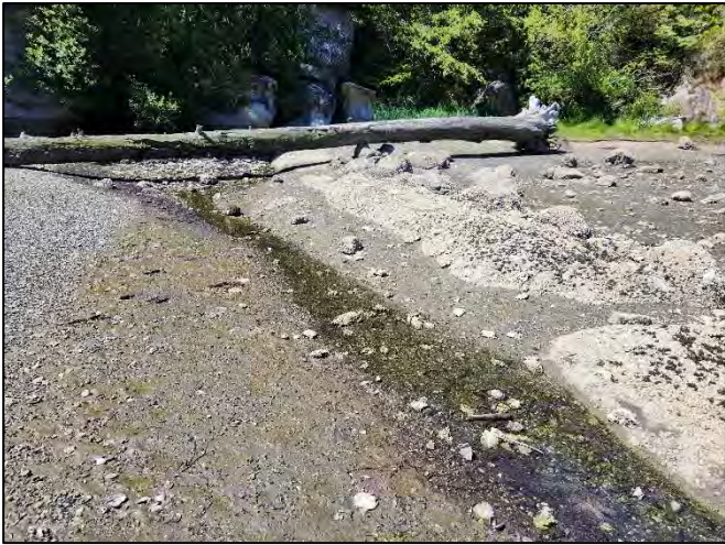
Photo 9: Closer view of flow channel conditions through upper tidal area.
