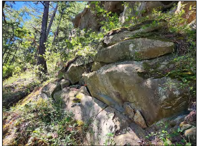
Photo 10: Fractured area of sandstone outcrop with loose rock exposed.
