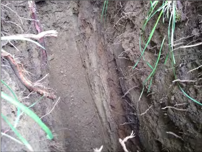
Photo 1: TP1 Subsurface; Fill over Glacial Drift and Till
