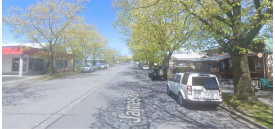
Figure 35. Existing conditions on James Street: 4 vehicle lanes, 2 parking lanes, no bicycle facilities
