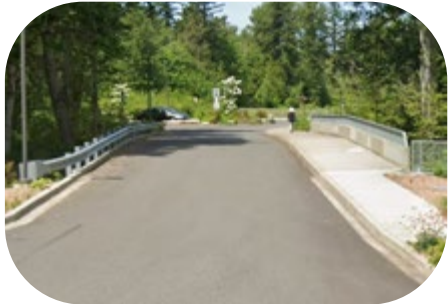
Stream Crossing Bridge Example from Julianna Park
