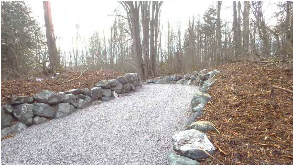
Photo 15. Typical Crushed Limestone Trail from Herrera's Design at Julianna Park, Bellingham, Washington.
