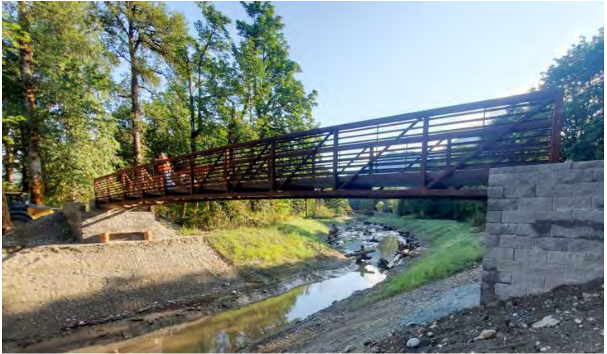
Photo 16. Example Pre-Fabricated Pedestrian Bridge from Herrera's Design at Pressentin Park, Marblemount, Washington.
