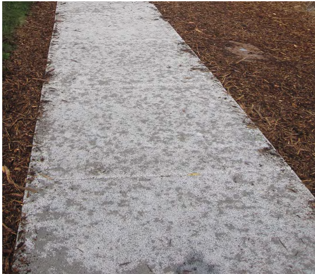
Photo 14. Pervious Concrete Trail, Westridge Place, Bellingham, Washington.
