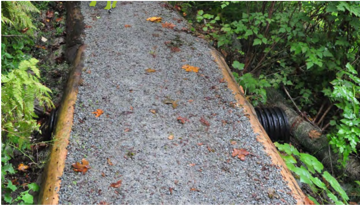
Photo 20. Example Culvert Installation Under a Trail.
