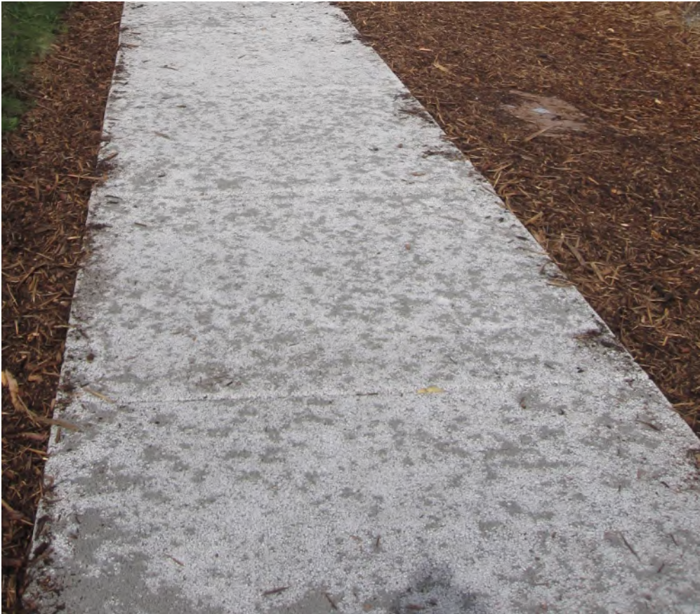
Photo 14. Pervious Concrete Trail, Westridge Place, Bellingham, Washington.
