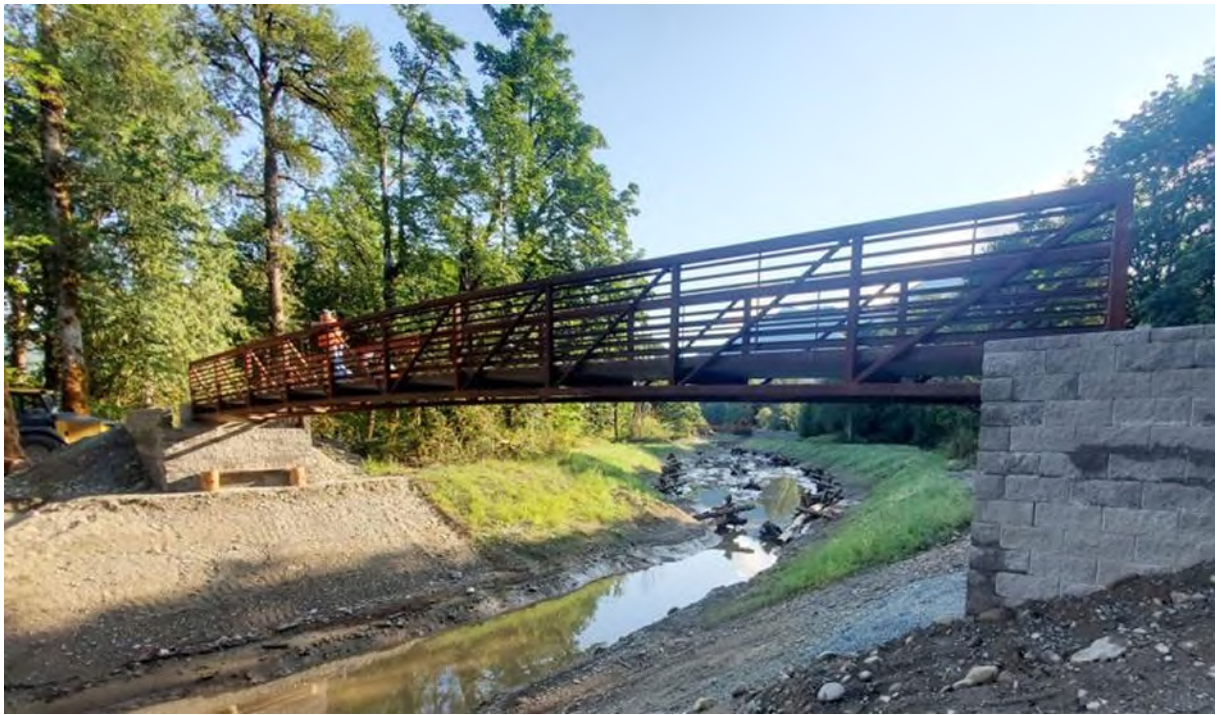
Photo 16. Example Pre-Fabricated Pedestrian Bridge from Herrera's Design at Presentin Park, Marblemount, Washington.
