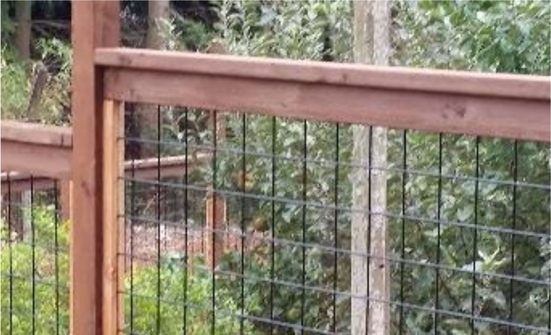
PHOTO 3: Note treated wood posts & top rail, cedar trim, and other details.
