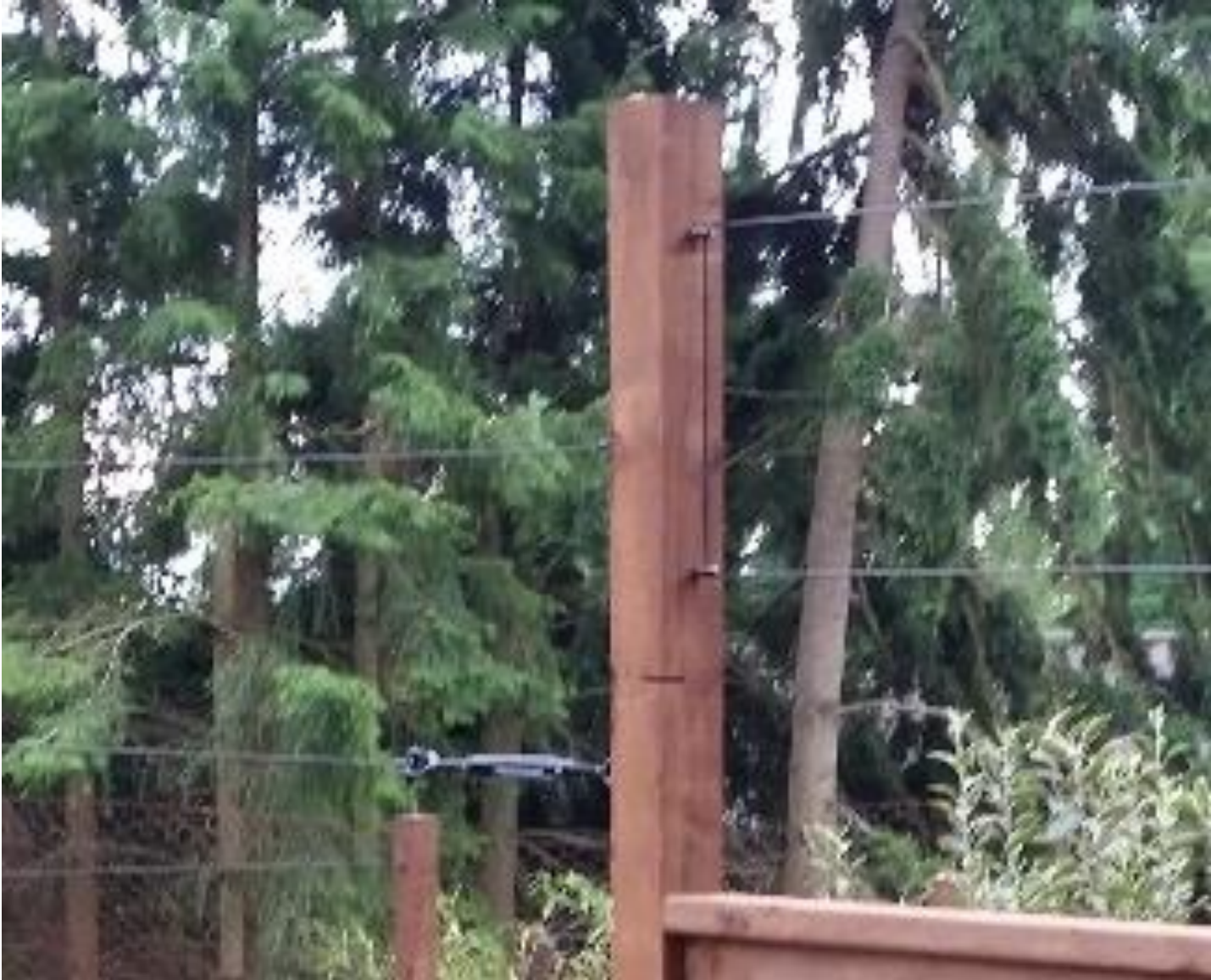
PHOTO 2: Note cable connections, tensioner, vinyl coated cable, and other details.
