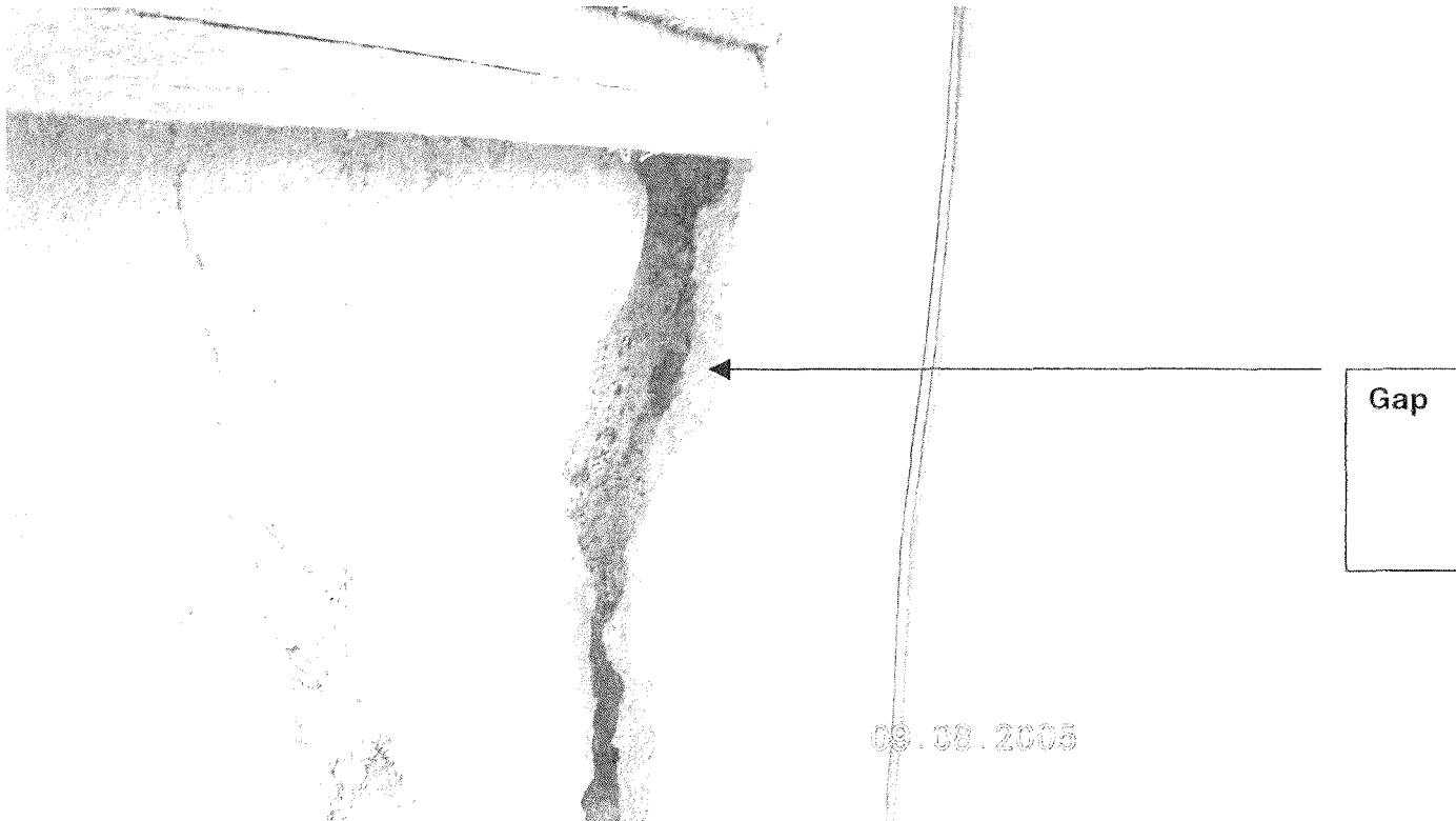
Crack in basement wall with gap where wall has pulled away from the retaining wall.
