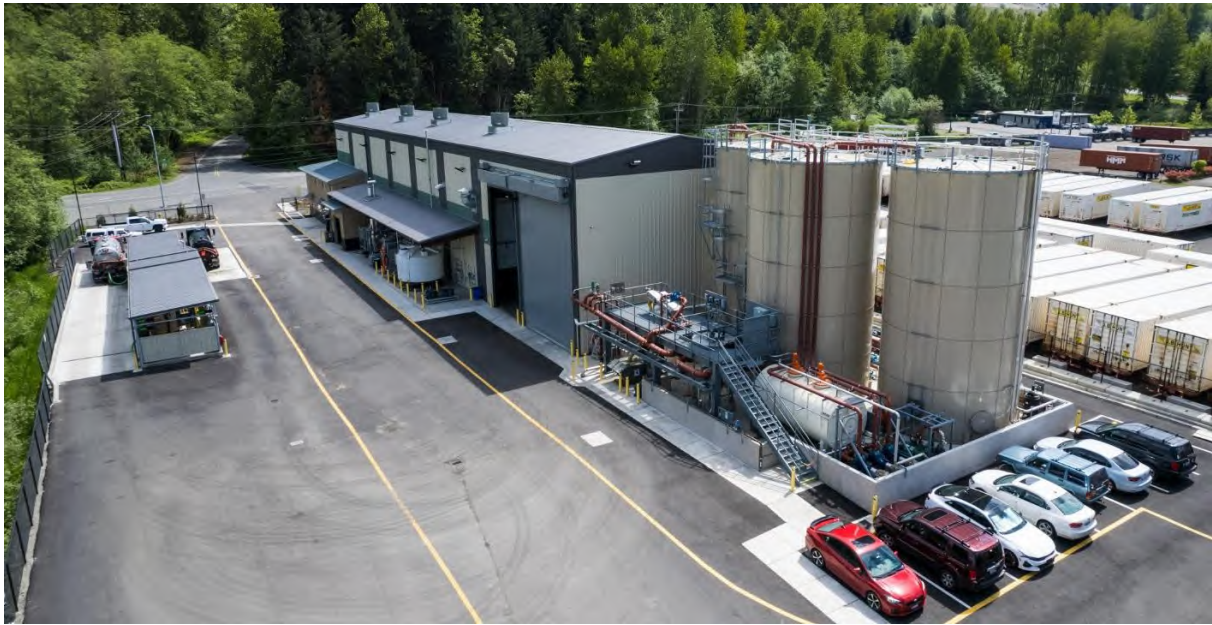
Sumner Septage and Biosolids Processing Site
