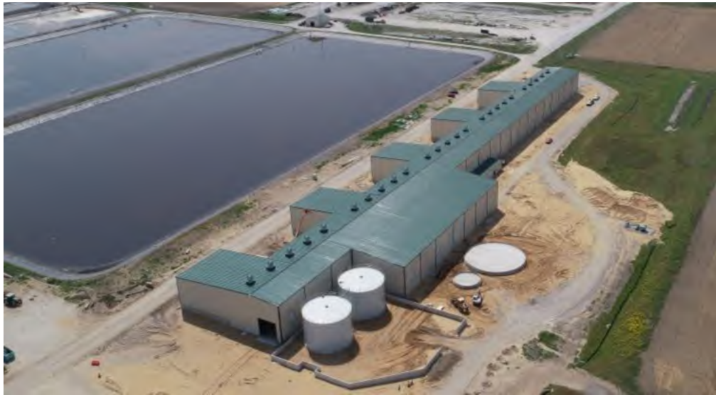
Varcor Building at a Dairy Farm in Northern Indiana
