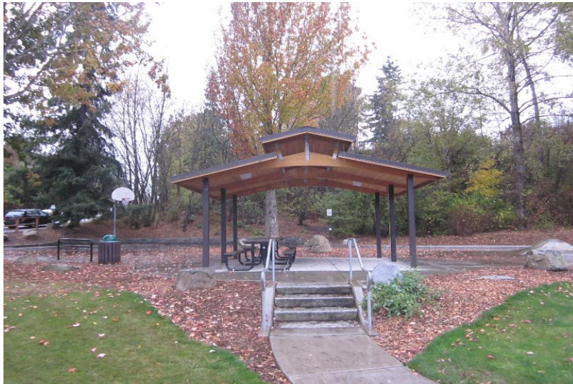
Franklin Park Picnic Shelter
