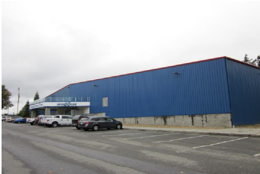
Exterior View - Civic Complex Sportsplex, East Elevation
