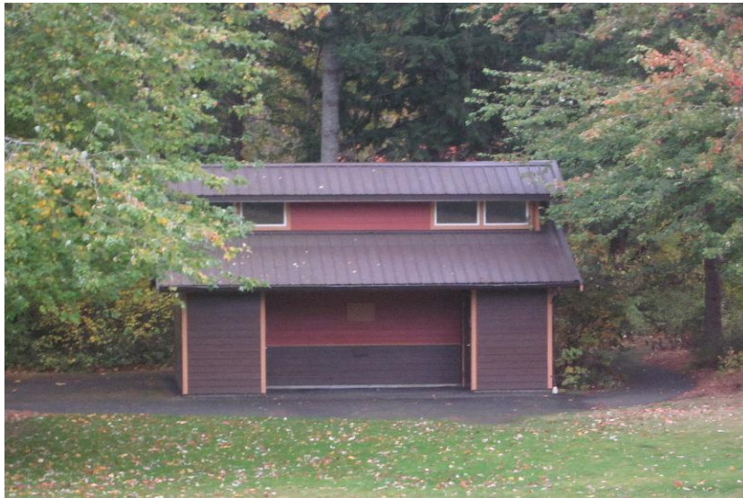
St Clair Park Restrooms
