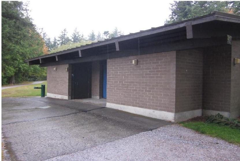
Lake Padden Park Playground Restroom
