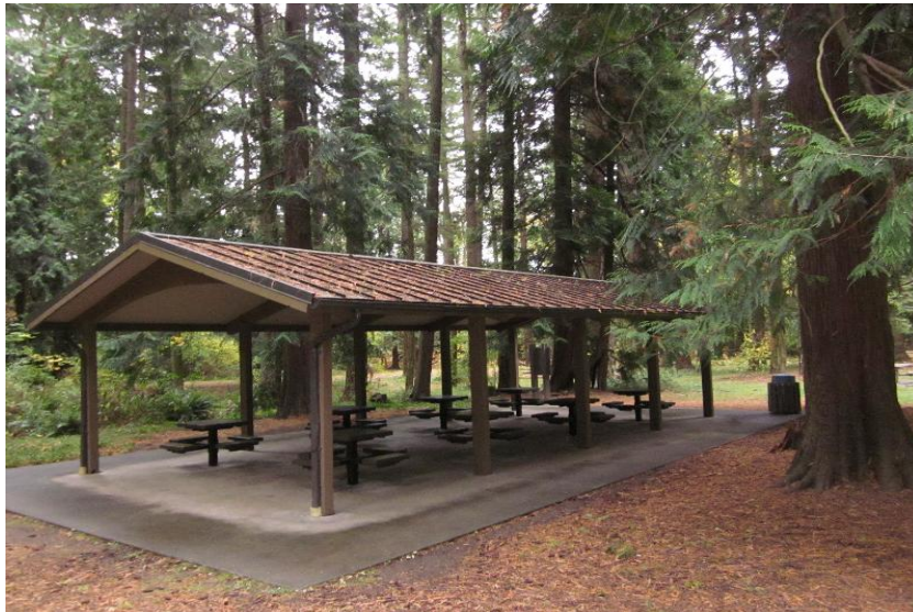
Cornwall Park South Picnic Shelter
