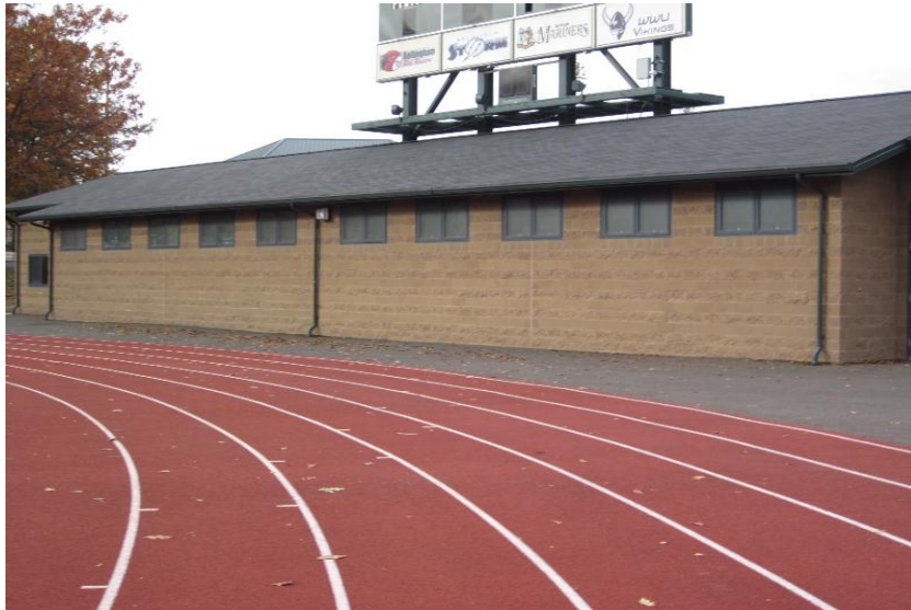
Civic Field Free Standing Locker Room
