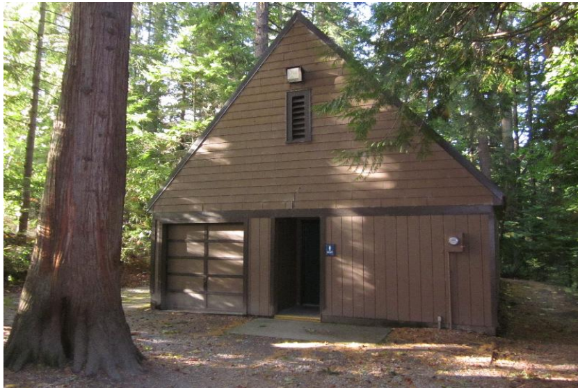
Paint (Exterior) Renewal
