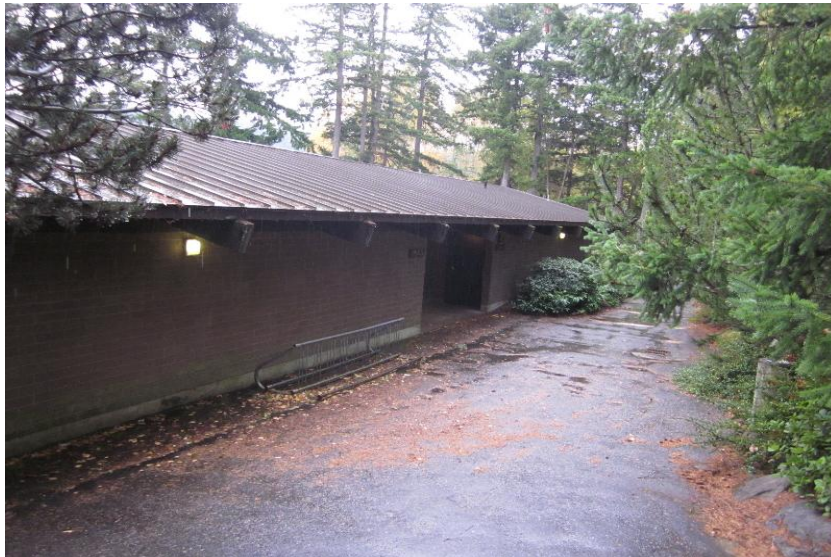
Lake Padden Park Bathhouse Restroom
