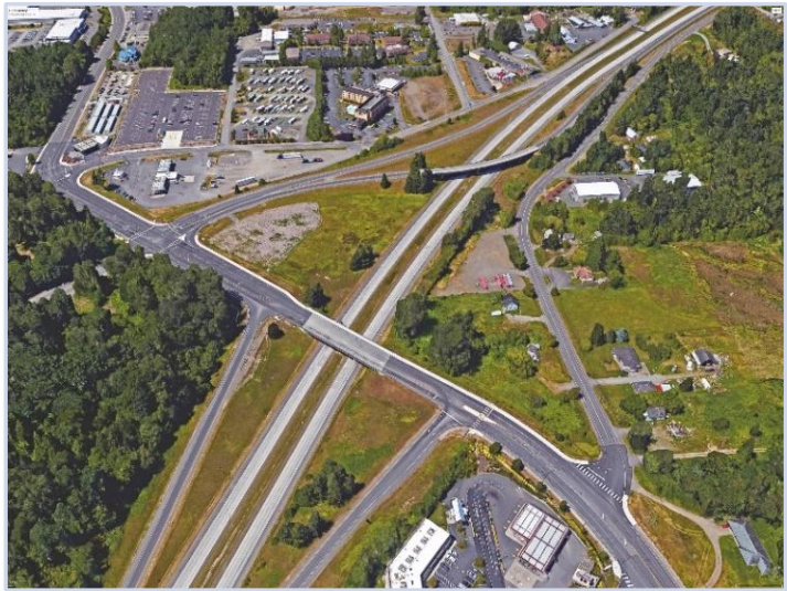
I-5/Bakerview Road Interchange
