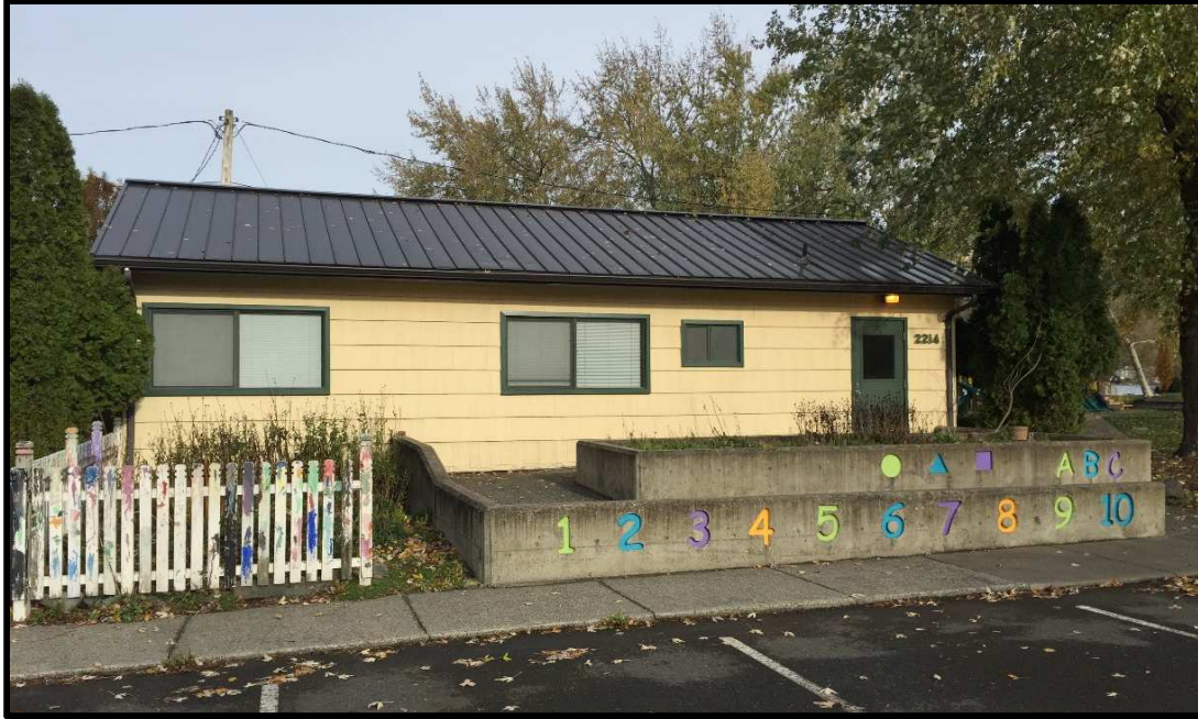
Building exterior from parking lot
