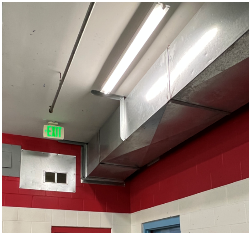
Figure 2.3-7: Furnace Ducting & Return Grille
