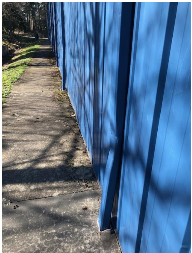
Existing downspouts bent, dented or corroded through. Damaged gutters to be replaced and connected to existing stormwater drainage system.
