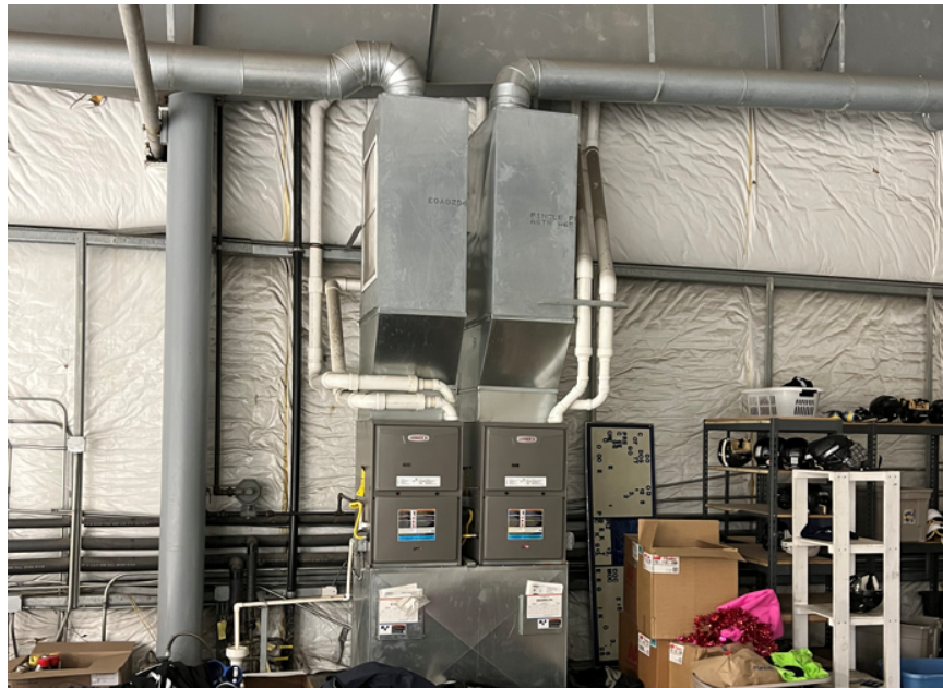
Figure 2.3-5: Ducted Furnaces – Dressing Rooms, Restrooms, Kitchen Areas
