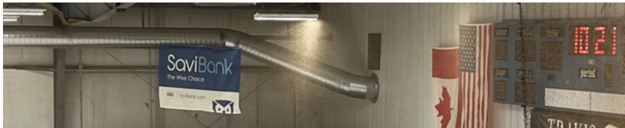
Figure 2.3-10: Dehumidifier Supply Ducting & Return Grille
