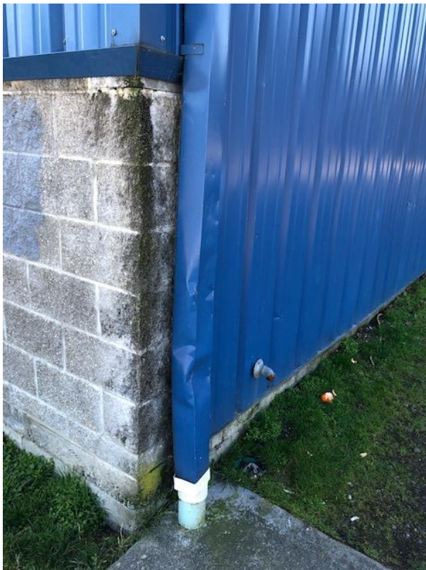
Existing downspouts bent, dented or corroded through. Damaged gutters to be replaced and connected to existing stormwater drainage system.
