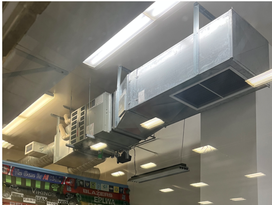
Figure 2.3-3: Gas Furnace w/ DX Coil – Ticket Office Area
