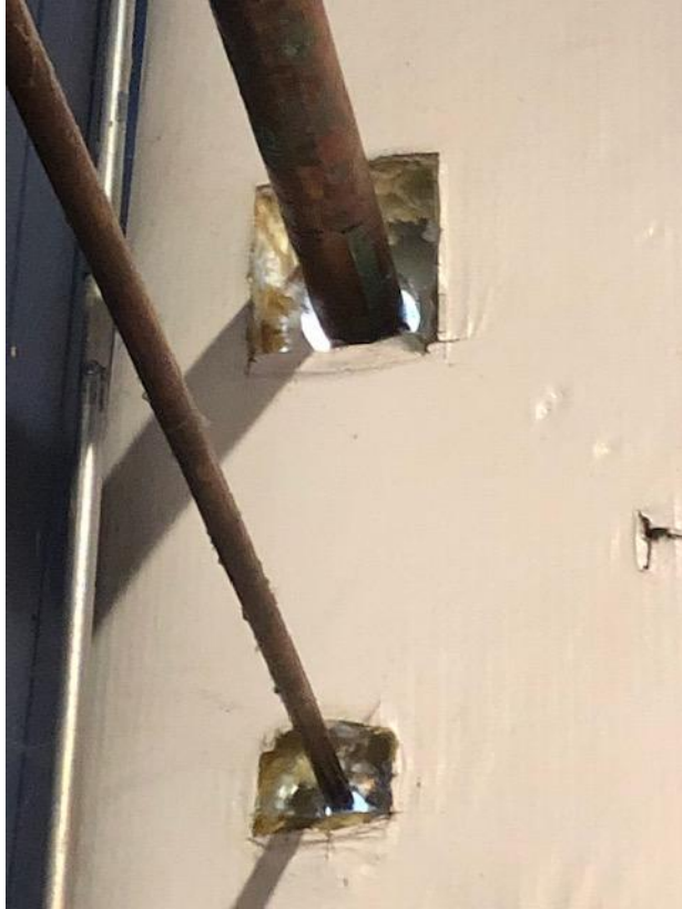
Proper flashing and weathersealing is needed at southwest exterior wall penetrations.
