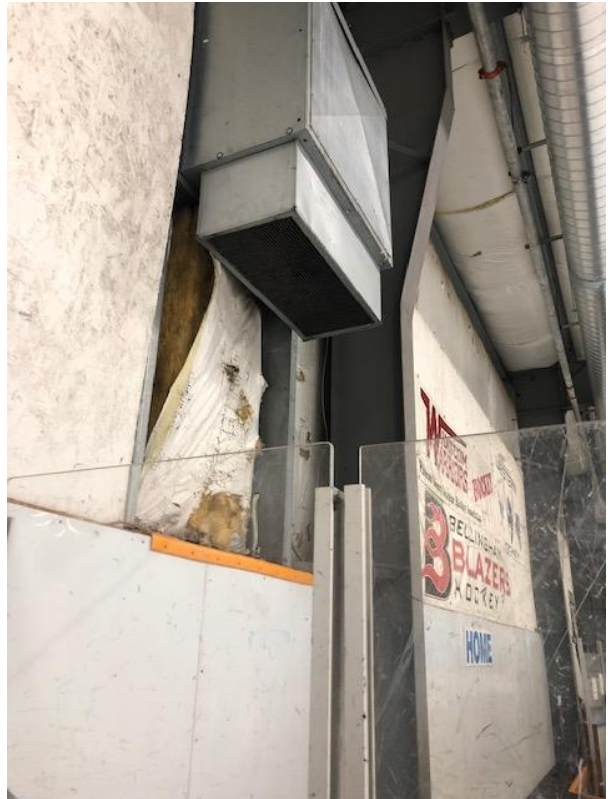
Insulation and vapor barrier damage on south wall of ice arena.
