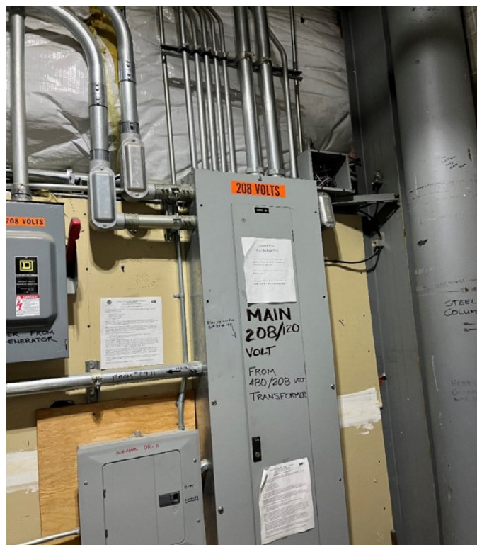
Figure 2.4-2: 208V Electrical Distribution Equipment
