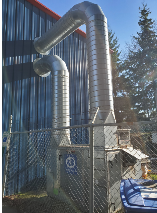
Figure 2.3-9: Dehumidifier Serving Ice Rink Area
