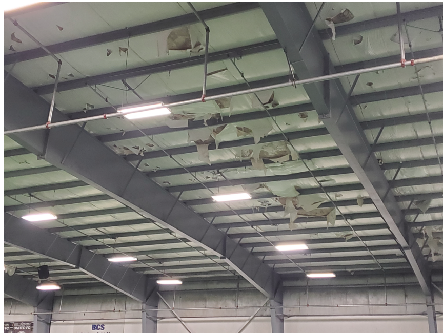
Figure 1.2-2: Water Damage to Insulation (Soccer Field Area)
