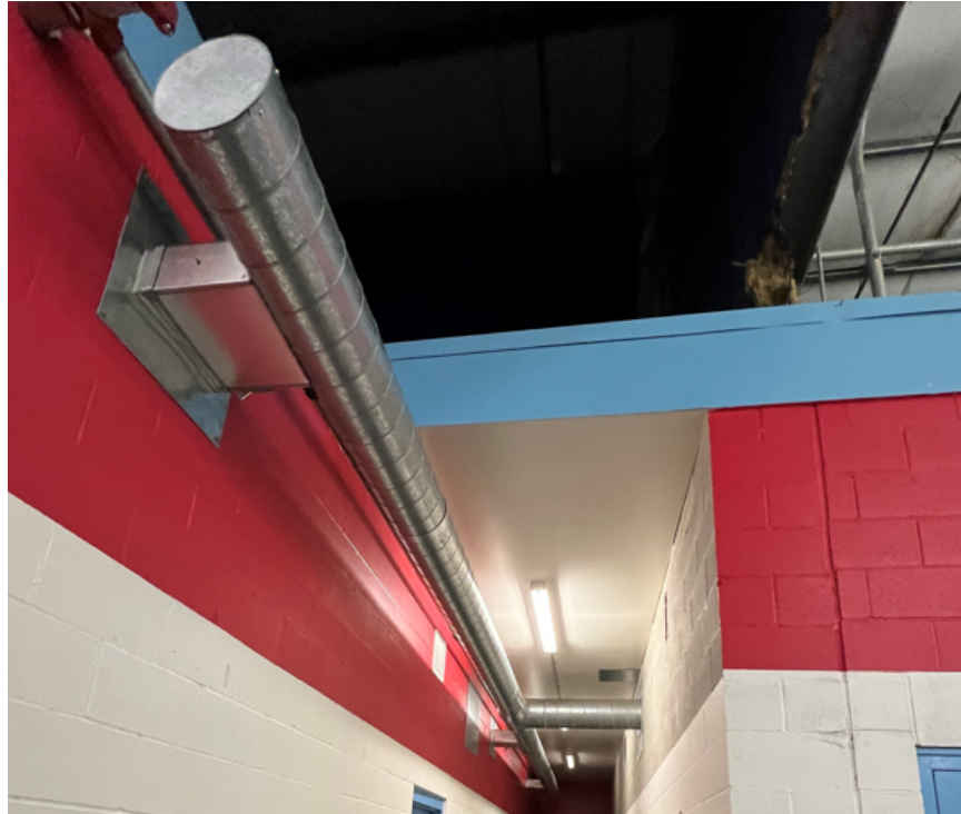
Figure 2.3-6: Furnace Ducting to Dressing Rooms
