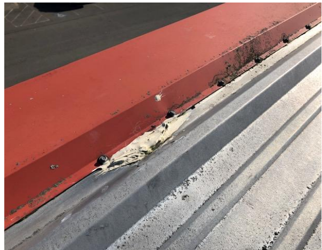
Many flashings are loose or bent and do not provide a weather tight seal. Temporary caulking has been applied in many locations.
