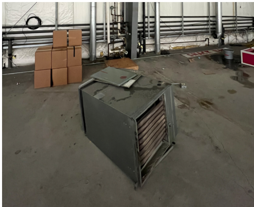
Figure 2.3-1: Gas Unit Heater – Ice Rink Area
