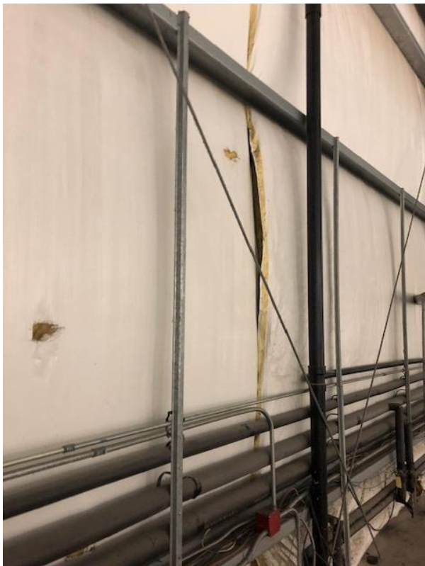
Failed seams in vapor barrier above locker rooms.
