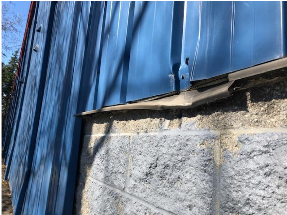
Repair damaged metal siding and flashing at Southeast corner of building. Gently clean and remove paint from CMU and reseal with anti-graffiti and weather protective coating.
