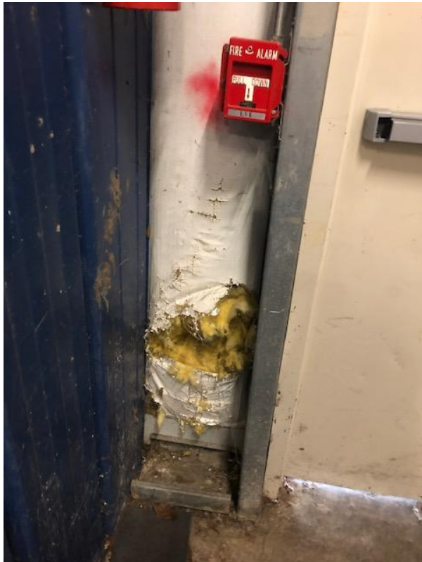
Insulation and vapor barrier damage at emergency exit on the west end of the ice arena.
