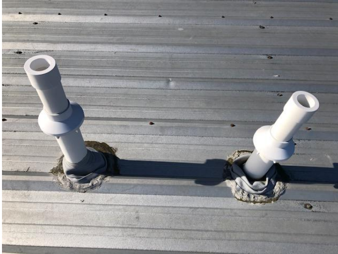
Pipe penetration boots and seals have failed. Replacement required.
