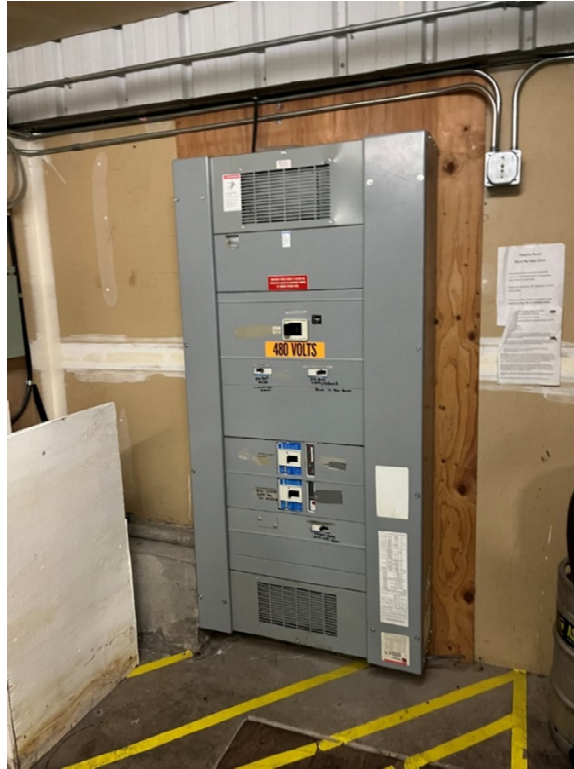
Figure 2.4-1: 480V Electrical Service Entrance Distribution Board
