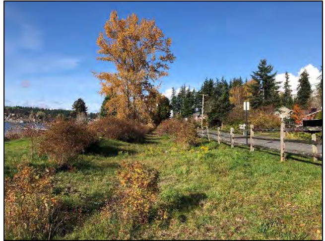
Photo 4: Conditions at the south end of the existing bioswale feature, looking North. (11-10-21)
