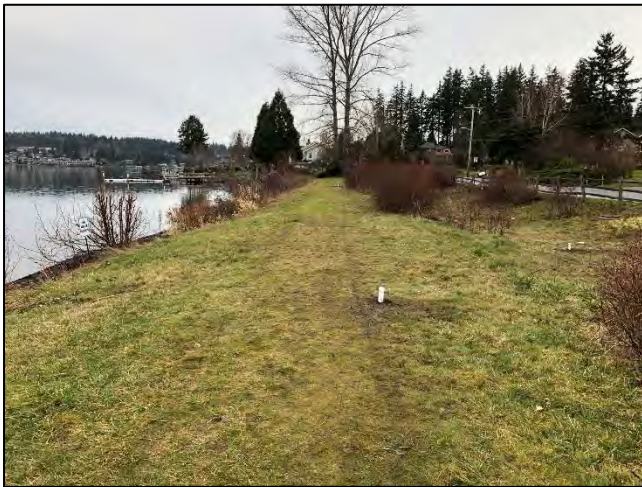
Photo 9: Conditions at boring location B1 at the south end of the berm feature, looking North. (2-8-22)
