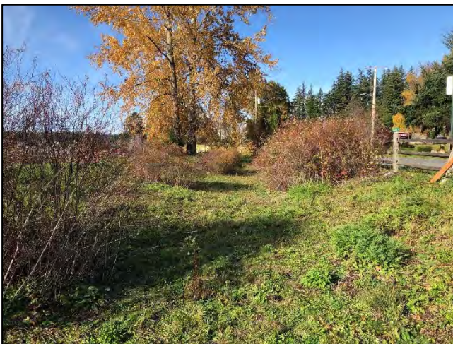
Photo 5: Conditions at the center of the existing bioswale feature, looking North. (11-10-21)
