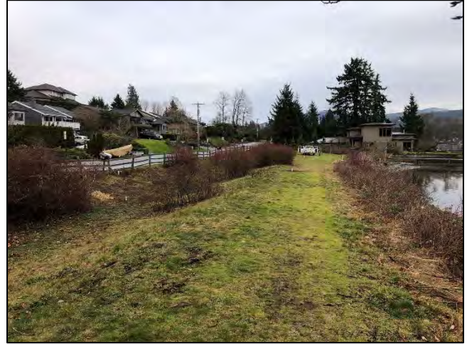
Photo 8: Conditions along the berm feature, looking South. (2-8-22)
