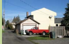
Maintain adequate side yard setback (no fire wall)
