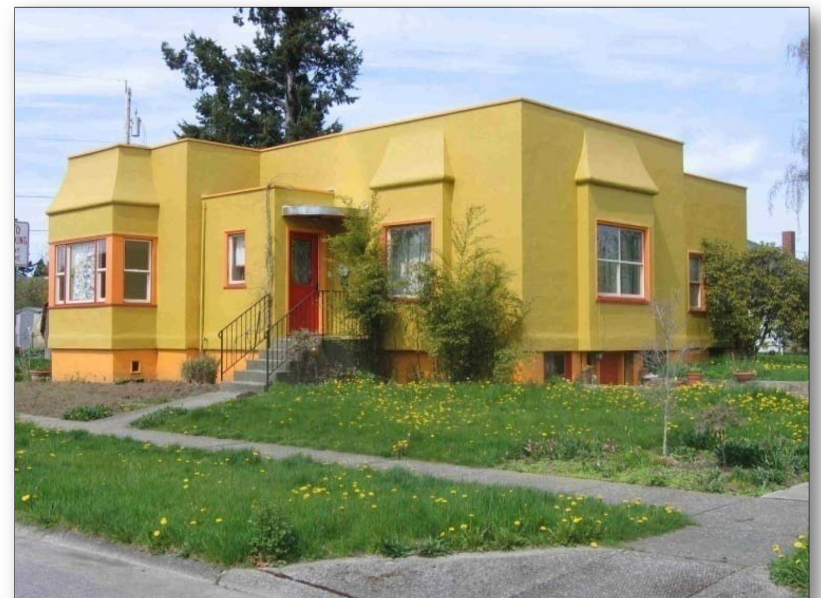
Example of a Duplex in Bellingham
