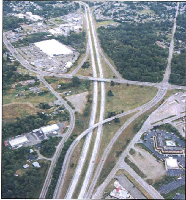
Exhibit PP1-E2: I-5/Bakerview Road Interchange looking south
