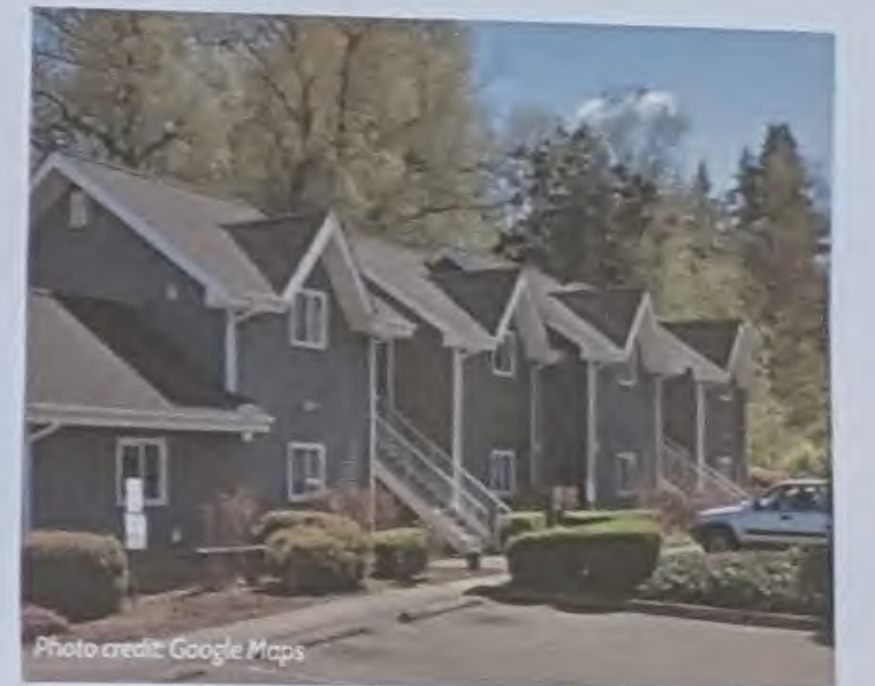
Willow Creek Apts Multifamily rental housing with 16 studio apartments for disabled adults. All units targeted to incomes <50% AMI.
