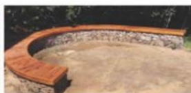
wood-topped gabion baskets
