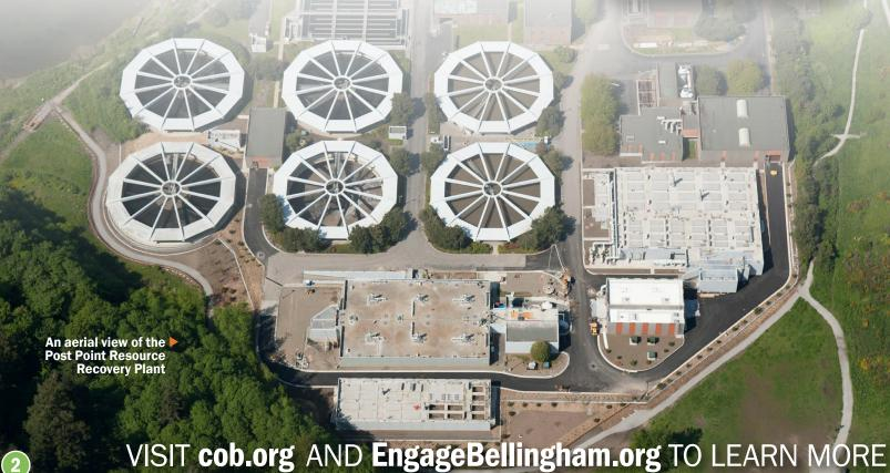
Post Point Wastewater Treatment Plant has been in operation for nearly 45 years. It includes two essential and related treatment processes: liquids and solids. In 2014, the City completed major upgrades to the liquid treatment process to improve performance, meet current regulations, and increase capacity for the future. As part of that project, the City also planned future upgrades to the solid's treatment process.
