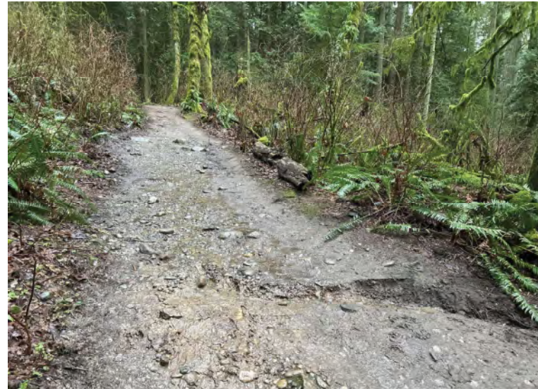
Erosion on unimproved trail- condition rating 4.
