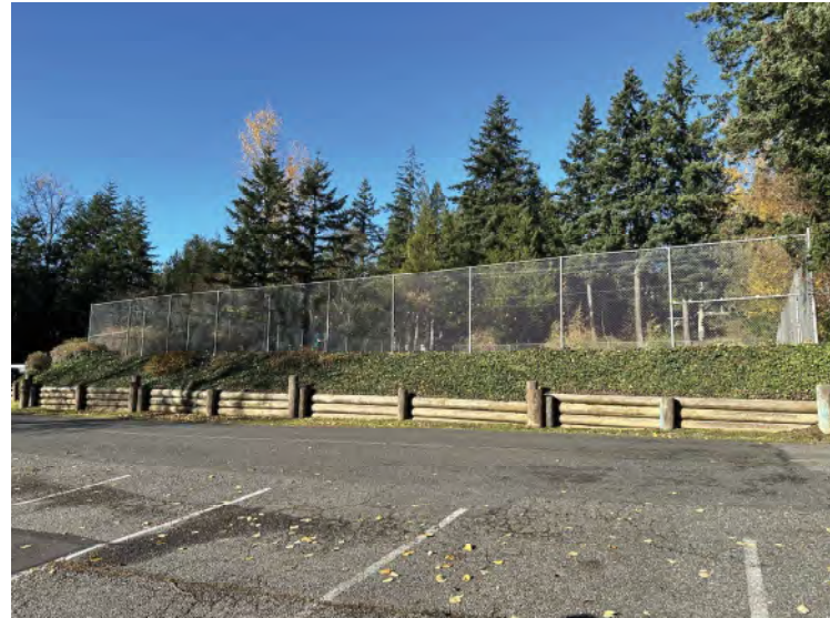
Tennis court as seen from parking lot. Condition rating 2.
