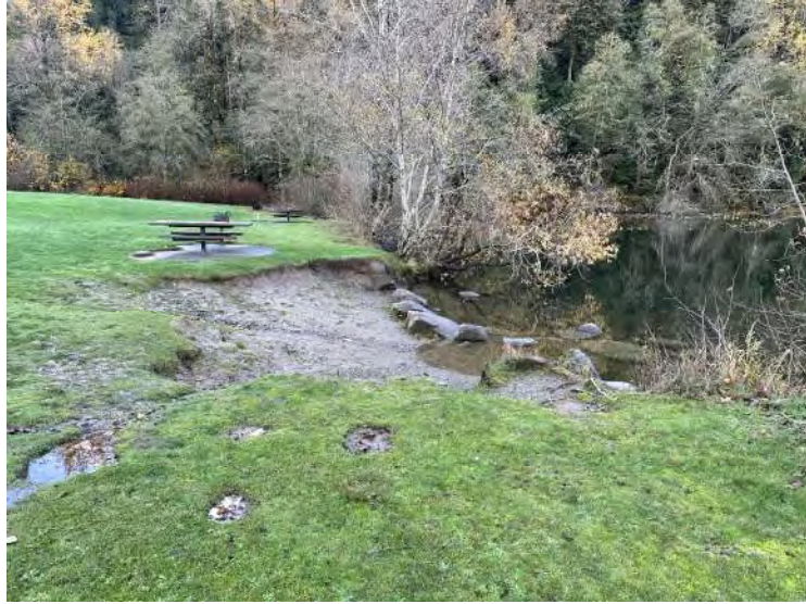
Shoreline erosion limiting water access.
