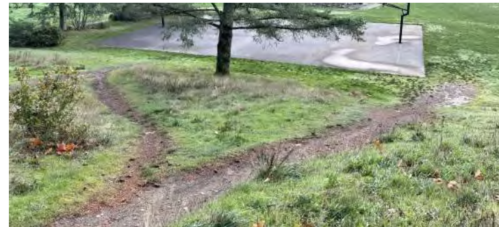
Footpaths contribute to slope erosion above basketball courts.
