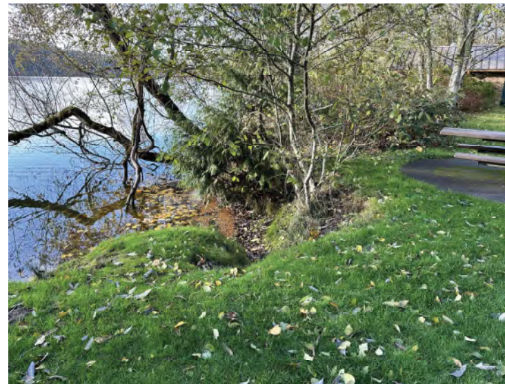
Bank erosion adjacent to picnic spot.
