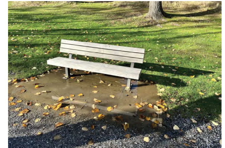
Bench pads do not allow for ADA seating adjacent.
