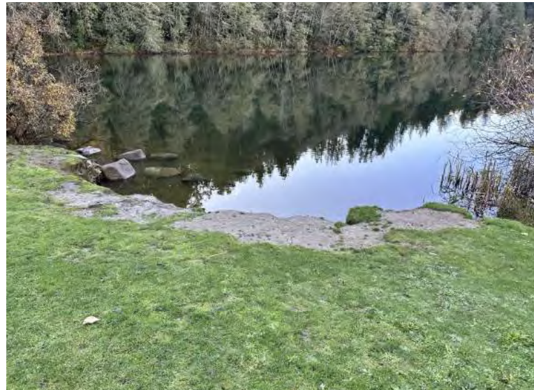
Shoreline erosion limiting water access.
