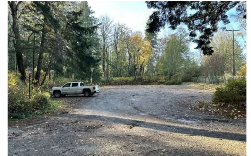
Horse trailer parking lot- condition rating 3.
