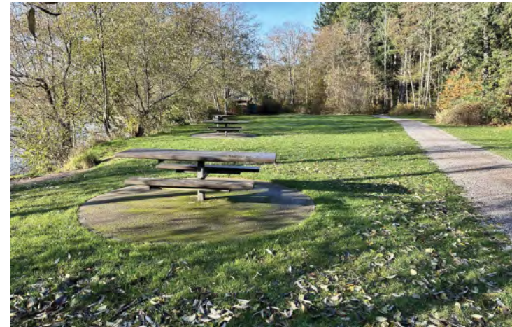
Picnic tables and concrete pads are not ADA compliant. Adjacent improved path is in good condition.
