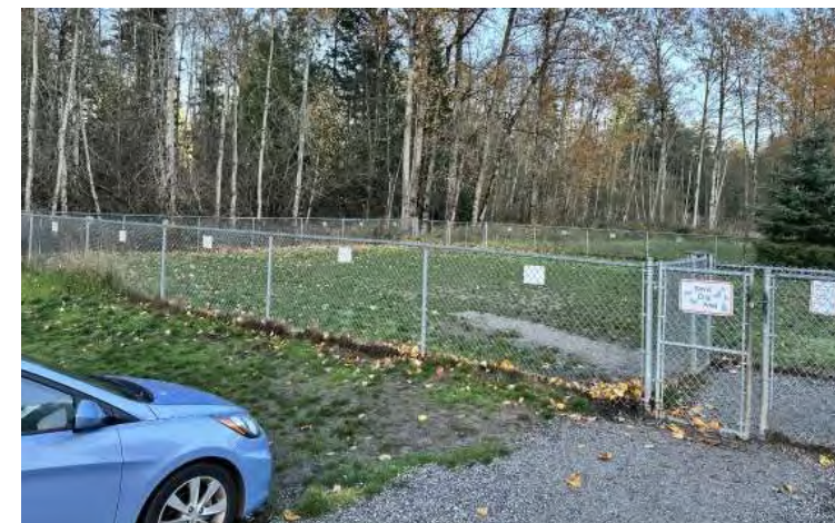
Dog park parking and fencing- condition rating 3.
