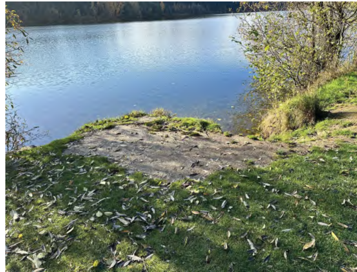
Bank erosion and compaction.
