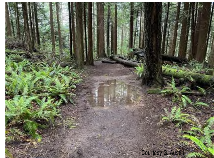
Standing water in unimproved trails- condition rating 4.
