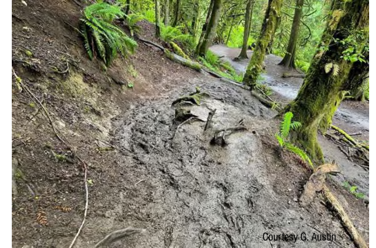
Unimproved trail with steep, muddy conditions with exposed roots- condition rating 5.
