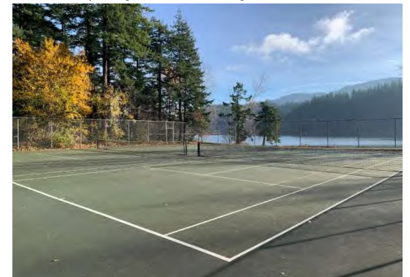
Tennis court- surface condition rating 3. Fence rating condition 2.
