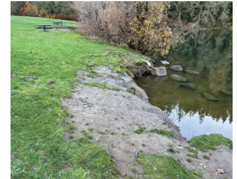
Figure 30. Eroded shoreline at the south end of the lake in Zone 9.
