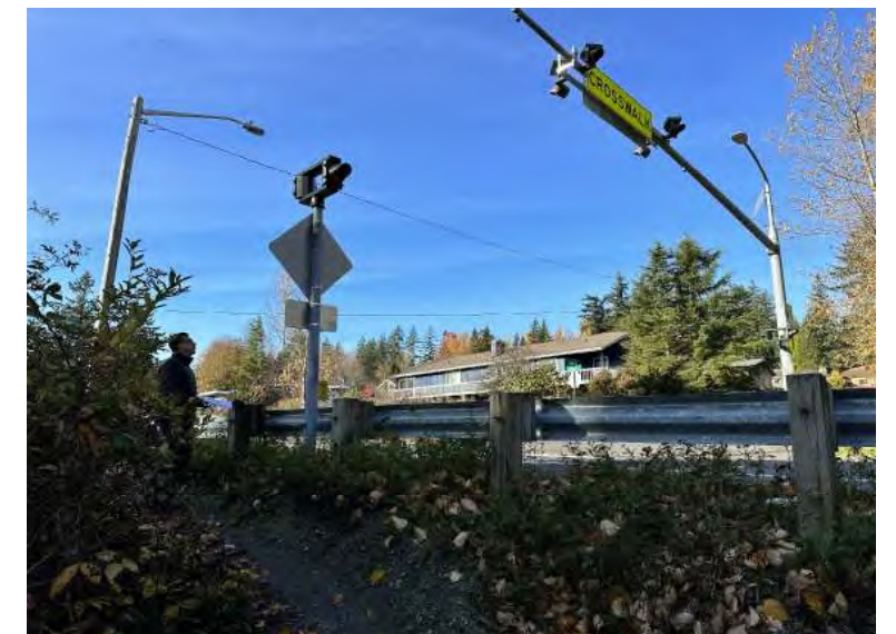
Informal pedestrian access from trail to Samish Way ties into pedestrian crossing. There is inadequate space for pedestrians to wait at crossing at the top of the trail.
