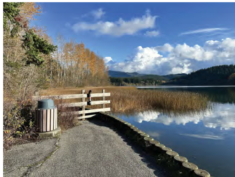
Fishing area bulkhead- looking south.
