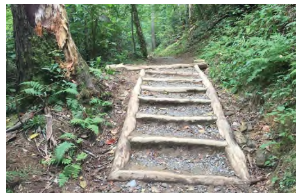
Figure 39: Wood stairs for steep trail sections
