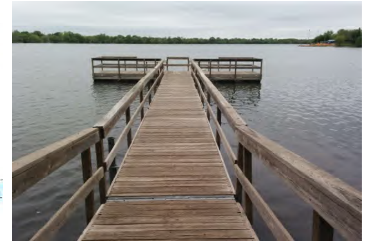
Figure 35: Fishing dock with railings
