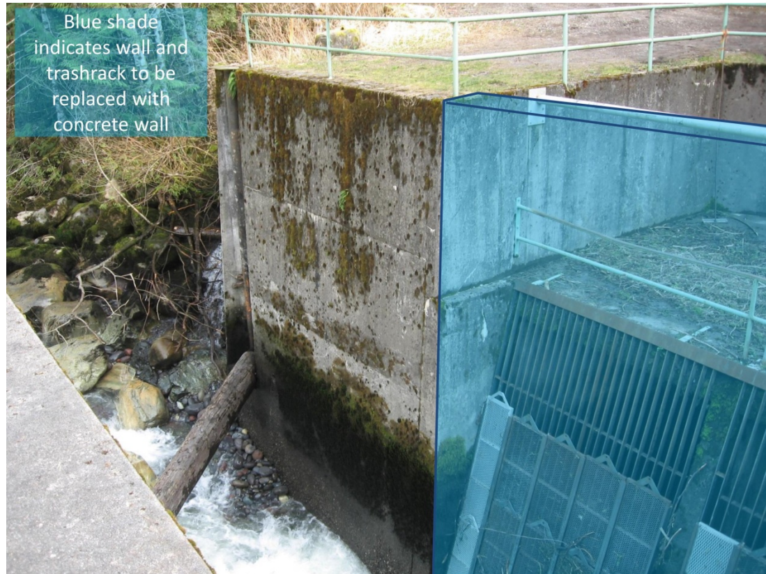
Figure 4-1. Alternative D - Existing Trashrack/Screen to be Removed and Replaced with a Concrete Wall.
