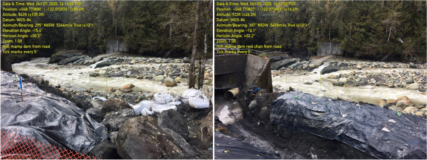
Photographs taken looking downstream from construction roadway
