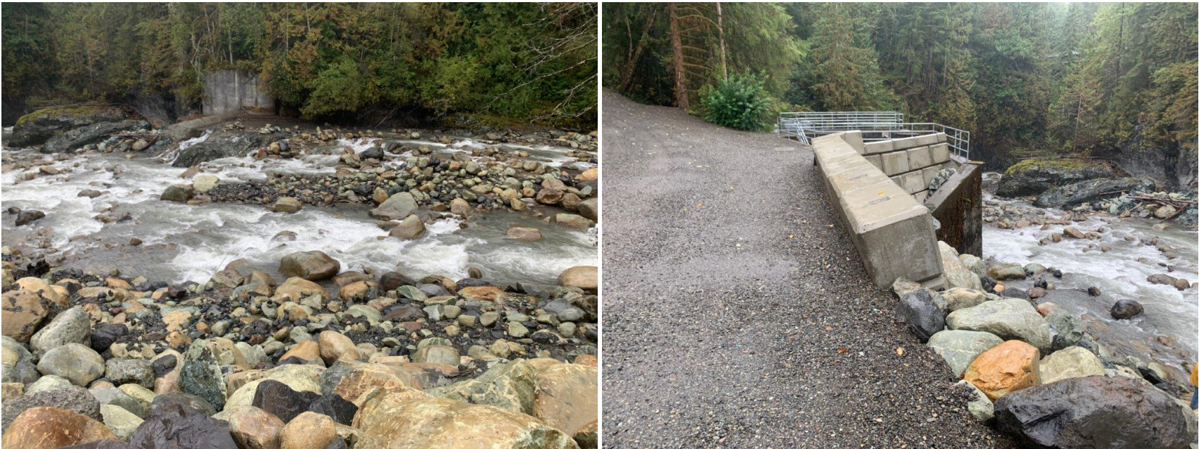
Photographs taken looking downstream from construction roadway
