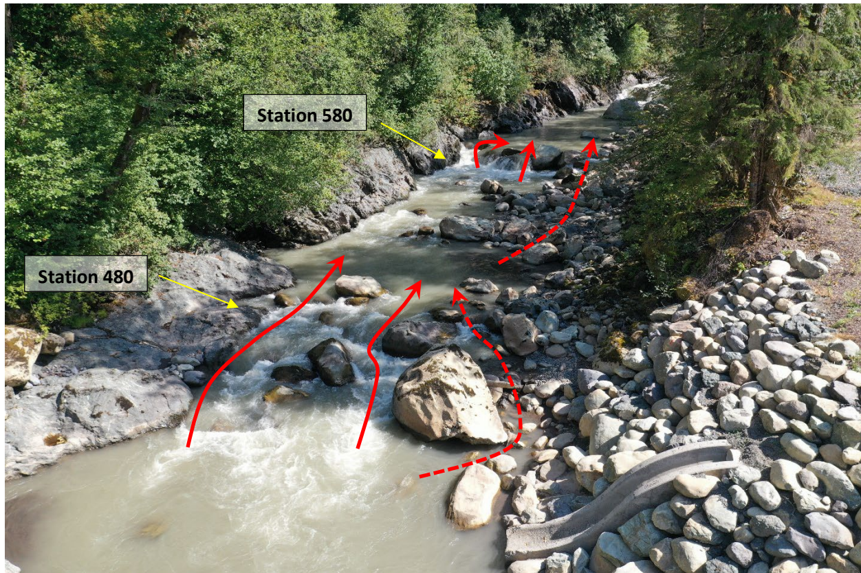
Figure 5.5 Likely passage routes at the observed flow at steps upstream of the fish outlet slide (September 2022). Solid lines = expected primary pathway during lower to mid-flow range; dashed lines = additional routes during mid- and higher flow range.
