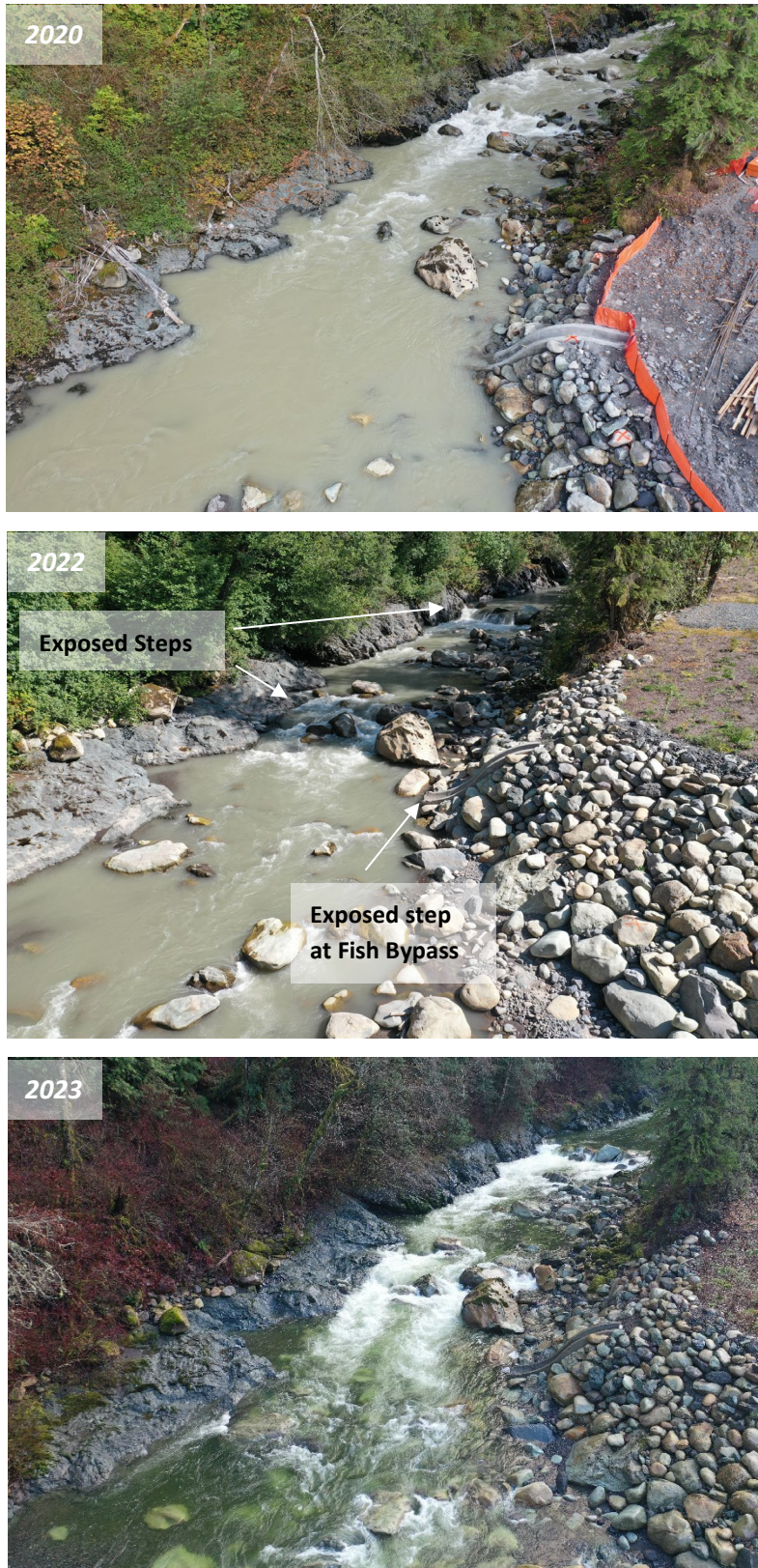
Figure 3.4 UAV oblique photos showing channel evolution at the pool outlet near Transect 400c between October 2020 (top, 225 cfs), September 2022 (middle, 152 cfs), and December 2023 (bottom, 410 cfs).
