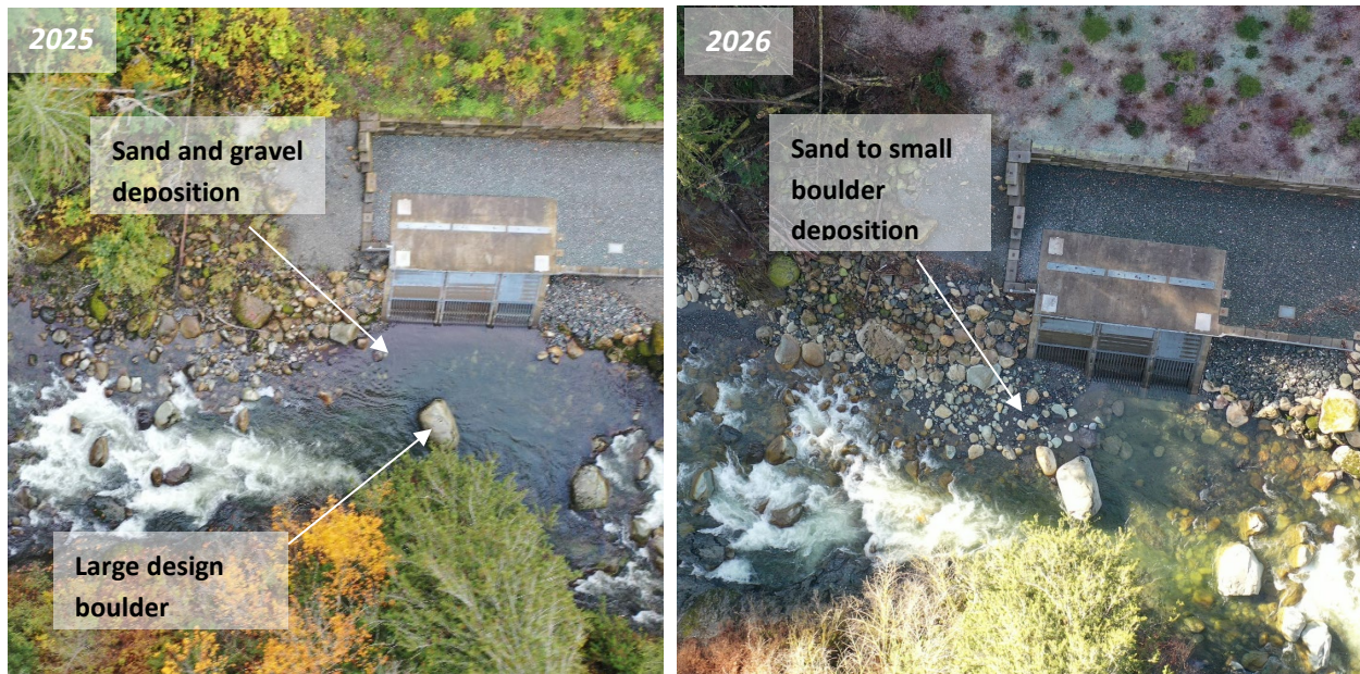
Figure 3.5 Comparison of the diversion structure in fall of 2025 (left) and spring of 2026 (right) (Photos: NHC)
