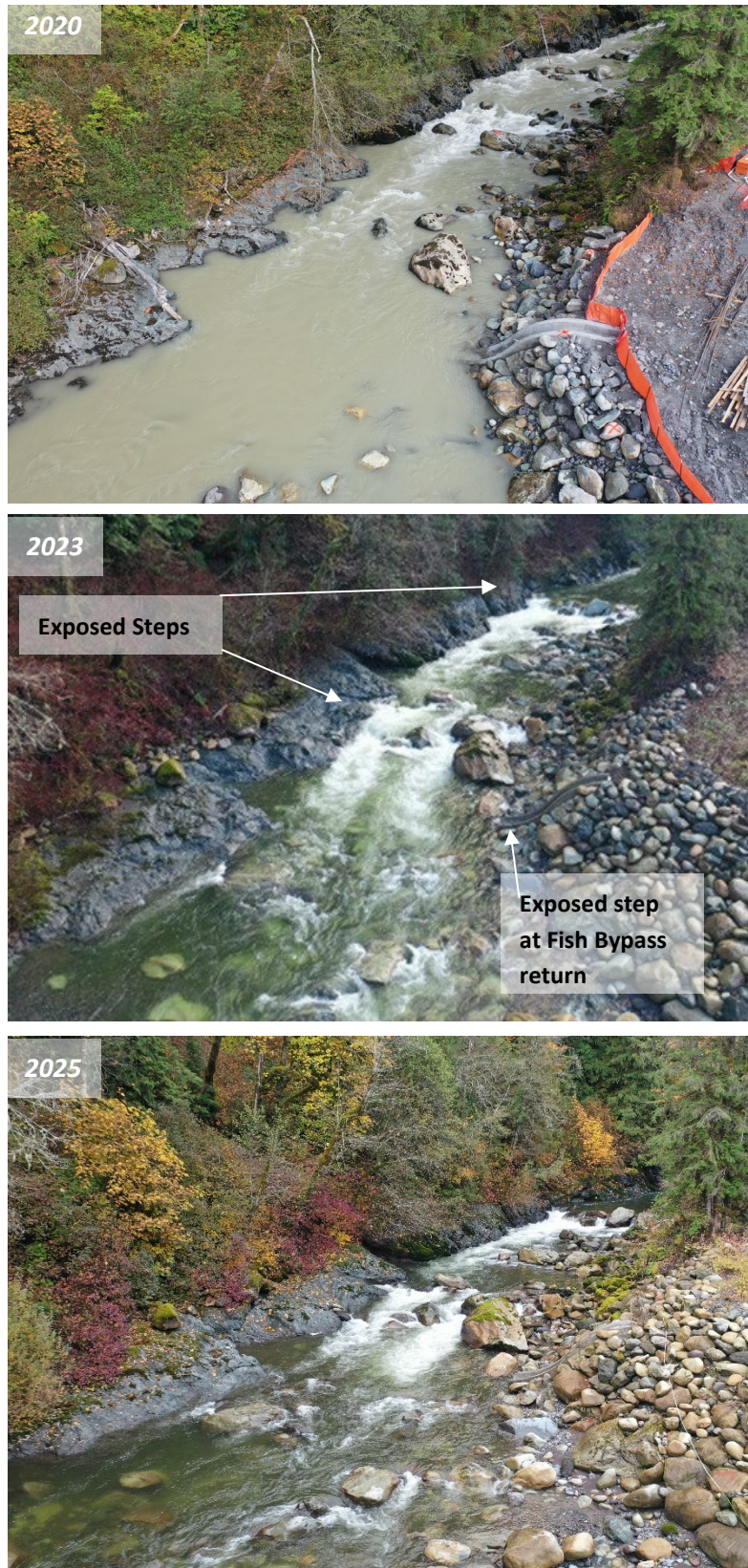
Figure 3.2 UAV oblique photos showing channel evolution at the pool outlet near Transect 400c between October 2020 (top, 225 cfs), December 2023 (middle, 410 cfs), and October 2025 (bottom, 225 cfs).
