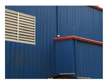
Downspout spills onto another roof. Recommend moving away from lower roof.
