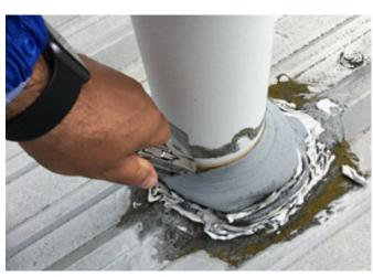
Sealant at pipe boots have failed, providing an inlet for mositure
