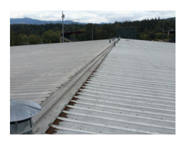
Debris has collected at both sides of the ridge. This condition can lead to moisture intrusion.
