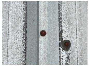
Many of the fasteners on the roof are rusted and will likely fail soon.
