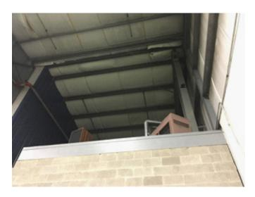
The insulation at the ridge on the West side of the building appears to be intact.
