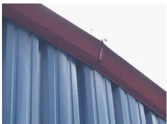
There is an opening in the edge metal; this condition can allow moisture into the roof system.
