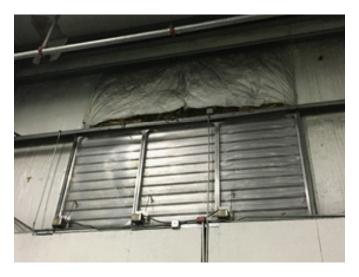
There is damage to insulation above some of the louvers.
