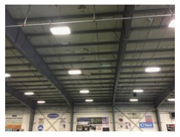
On the soccer side of the building, there are numerous locations where the insulation has failed.
