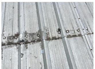
The laps in the roofing are not staggered, this can lead to moisture intrusion.
