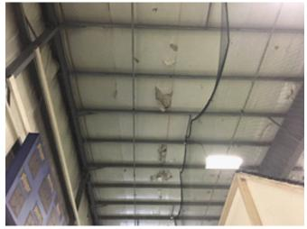
There are multiple locations of damage insulation in hockey side of the building.
