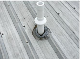
A majority of the pipe boots are sagging and collection of moisture, these conditions can lead to failure.
