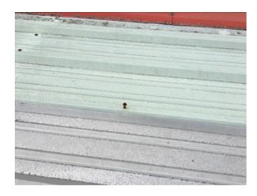
Some fasteners are backing out on the Northwest portion of the roof.
