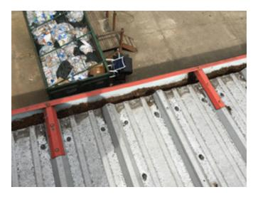
The standoffs for the gutter are installed over the roofing, creating an upslope lap. Combined with the hole from the fasteners, moisture will likely enter.
