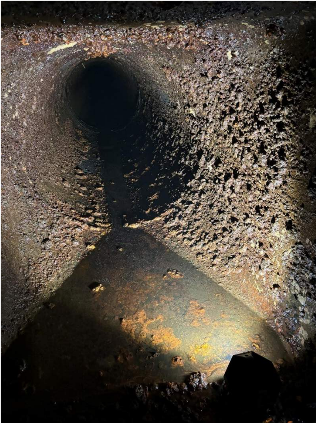
Exhibit 4-1. Tuberculation and Corrosion Product on South (Industrial) 48-inch Diameter Pipeline
