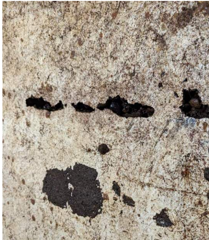
Exhibit 4-4. Outlet Well Cold Joint Line where Voids in Concrete Have Formed
