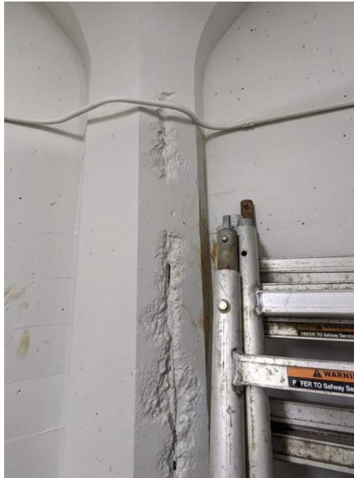
Exhibit 4-3. Spalled Concrete and Void Around the Exposed Reinforcing Bar
