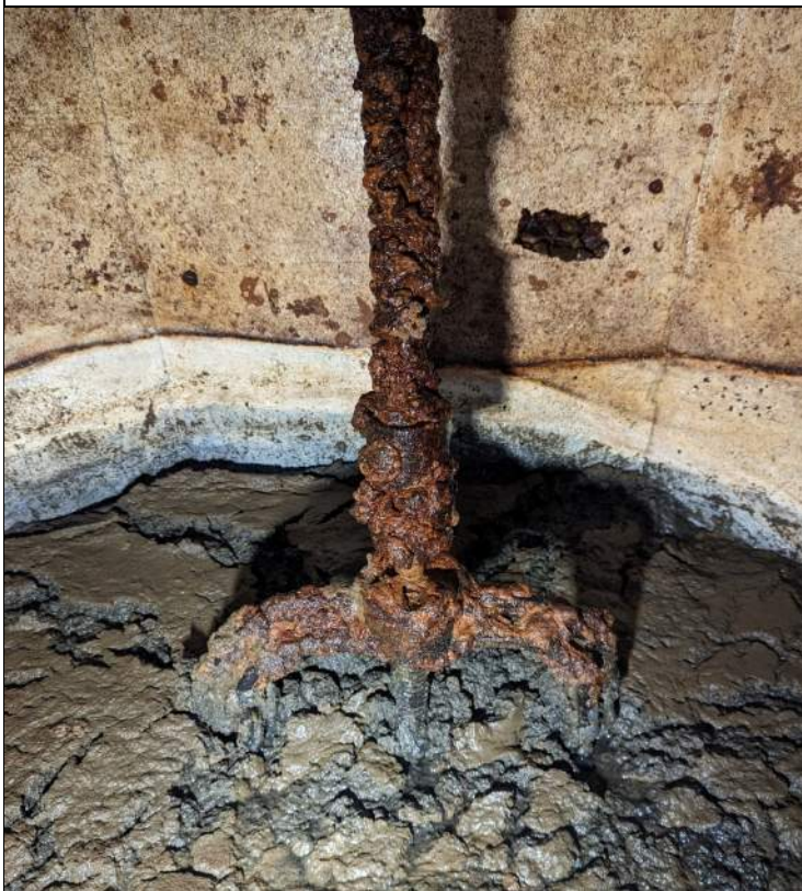
Photo #11: Mud Valve (Covered in Mud) and Valve Stem
