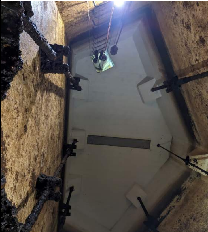
Photo #3: Ceiling at Outlet Well including Removable Gate Access Slot, Access Ladder and Gate Stems
