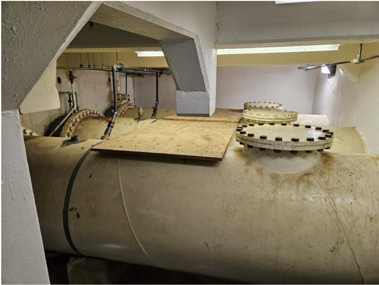
Exhibit 4-2. Discharge Pipelines in Chlorine Injection Room
