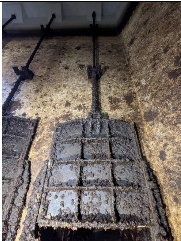
Photo #14: Discharge Pipeline Slide Gate (North)
