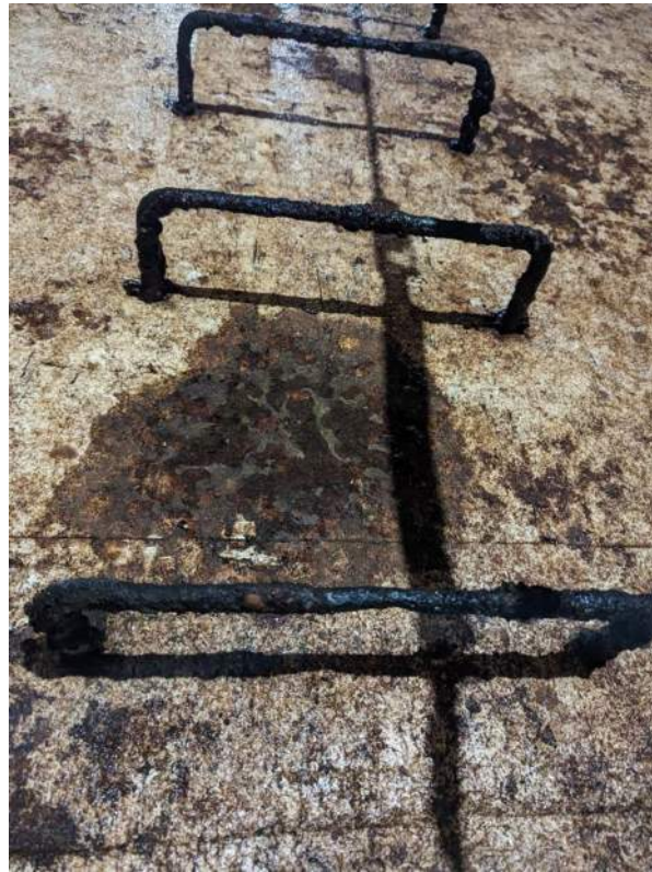
Exhibit 4-5. Ladder Access Rungs Show Severe Corrosion
