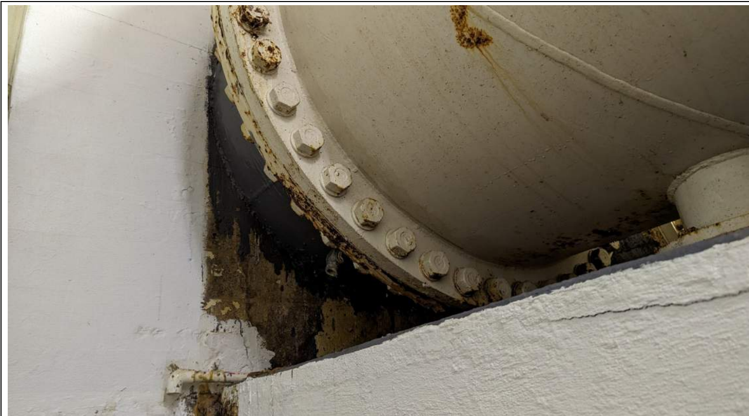
Photo #8: Discharge Pipeline in Chlorine Injection Room, Coating System (Black) added at Near Flange to Wall in 2013
