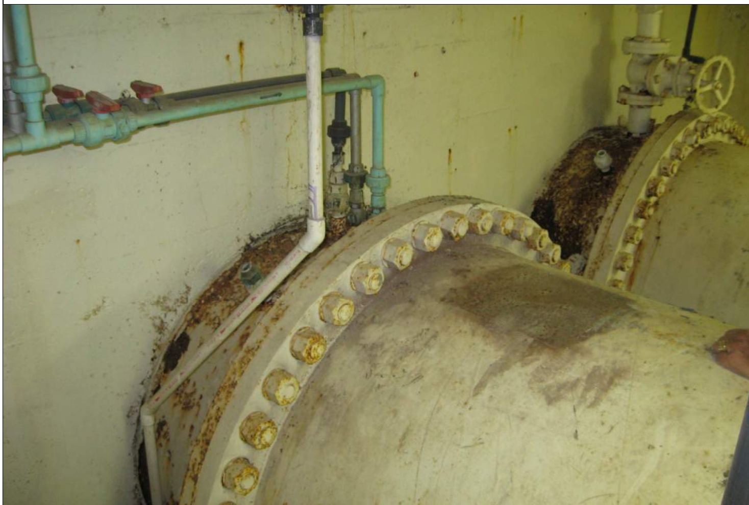
Photo #9: Discharge Pipelines in Chlorine Injection Room, Prior to Application of Coating System (Legacy Photo Circa 2012), Showing Extensive External Corrosion on Short Sections of 1940-Vintage Pipes.
