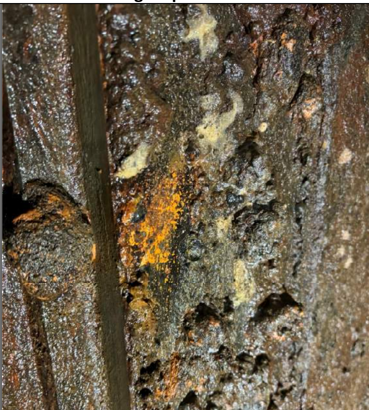
Photo #2: Tuberculation on Gate Frame at South (Industrial) Discharge Pipeline
