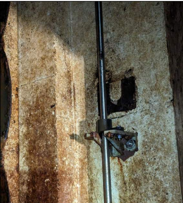
Photo #6: South Waste Well Gate Stem (Replaced early 2000s, Minimal Corrosion)
