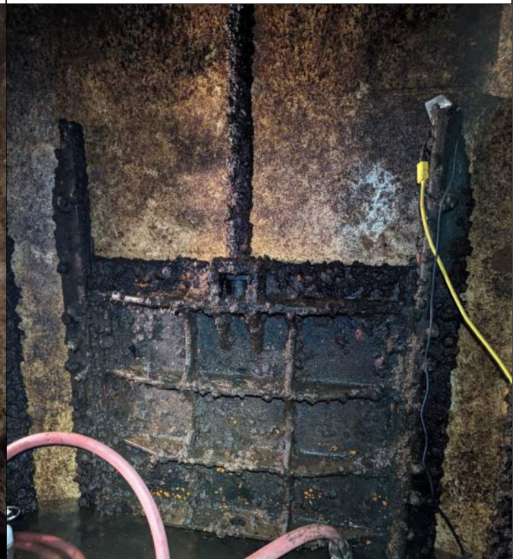
Photo #4: Intake Waste Well Slide Gate (Seized in Closed Position)
