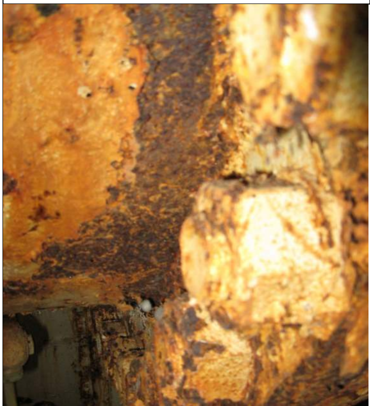
Photo #7: Corrosion on Discharge Pipeline Exterior and Flange in Chlorine Injection Room prior to Coating (Legacy Photo circa 2012)
