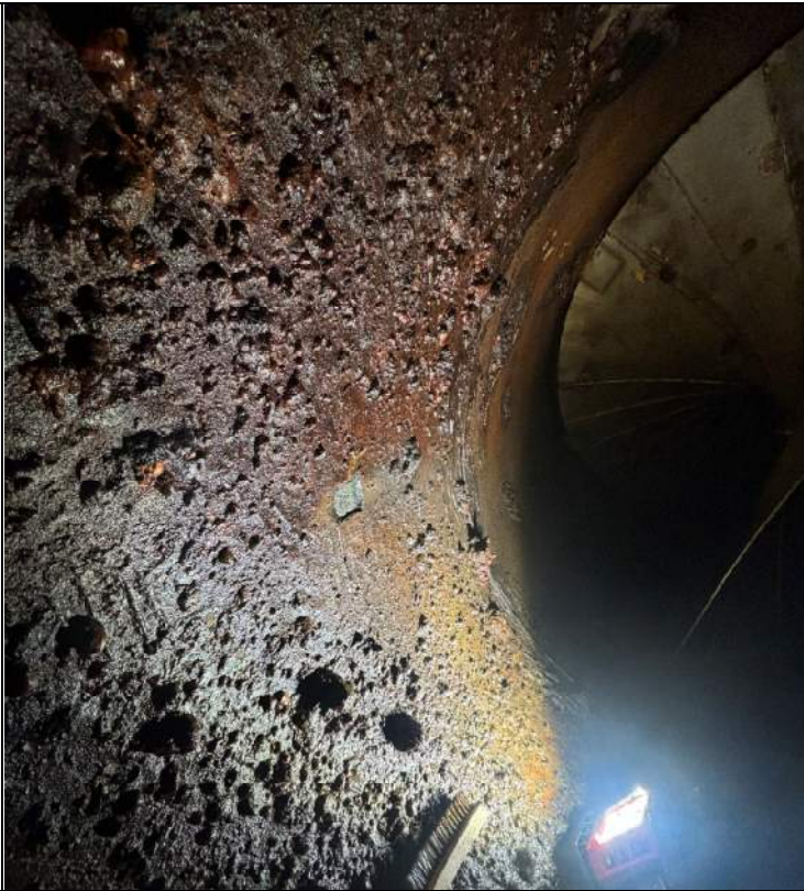
Photo #6: Thickness Testing Location in North Discharge Pipe
