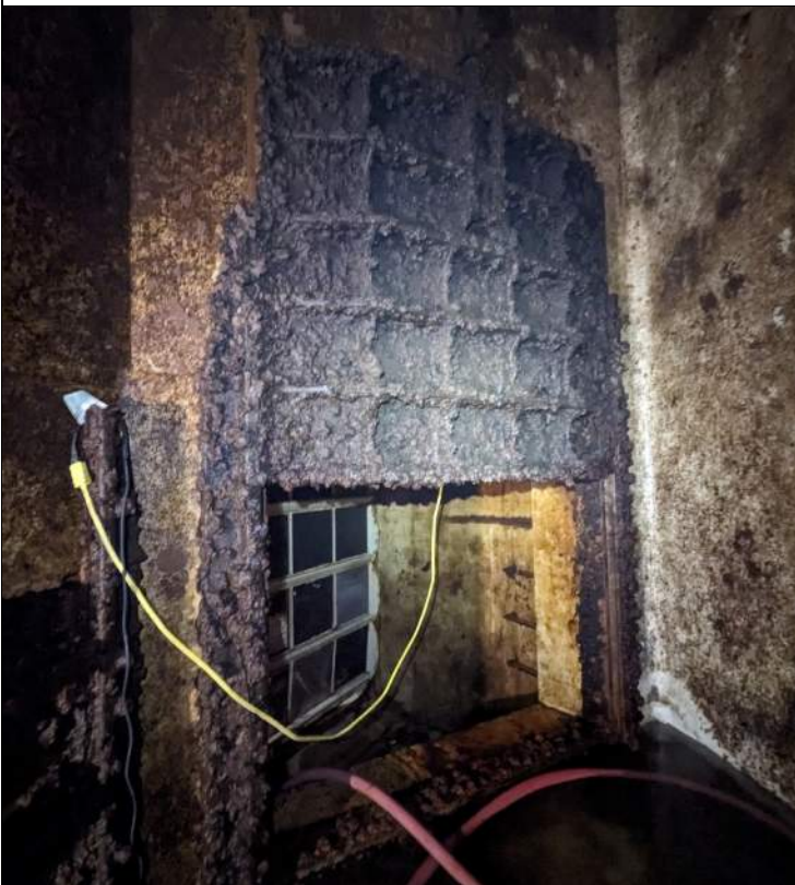
Photo #3: Intake Well North Slide Gate
