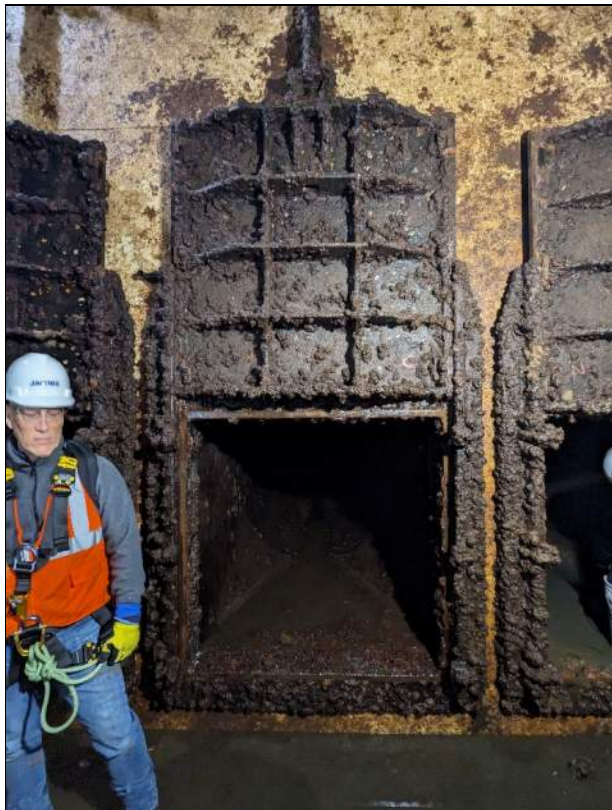
Photo #13: Discharge Pipeline Slide Gates
