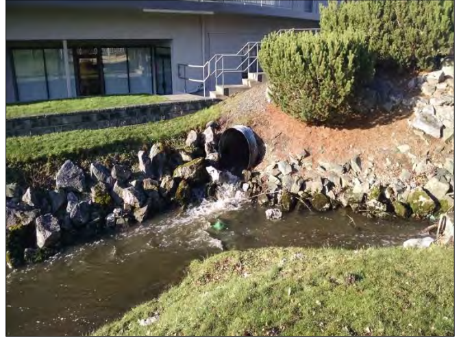
Photo 12: Culvert "mouth" of tributaries.
