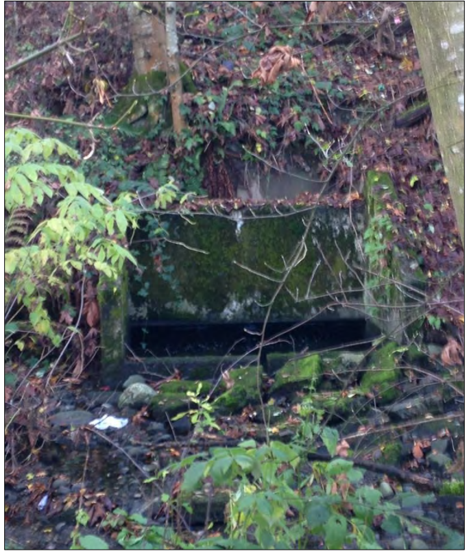
Photo 8: Relict stormwater feature.
