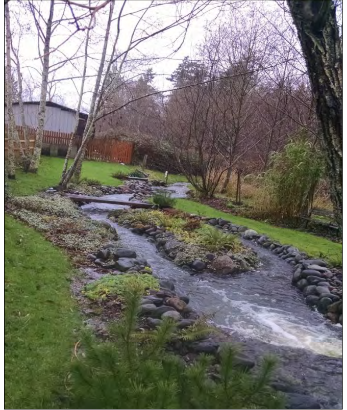
Photo 18: Channel modification on private property.
