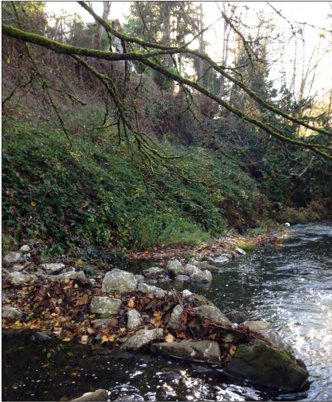
Photo 7: "Wing dam" with severe erosion in background.
