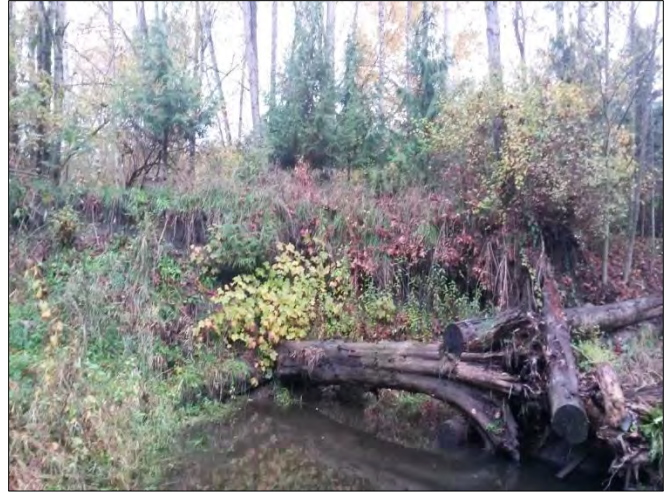
Photo 2: Installed LWD near mouth.
