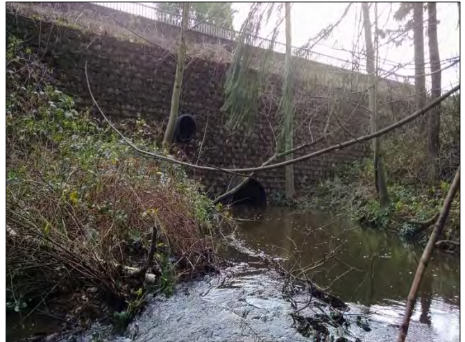
Photo 14: Culvert wetland near Bakerview Rd.
