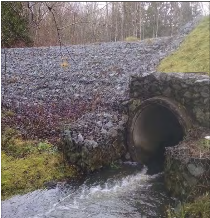
Photo 19: Stormwater control structure.
