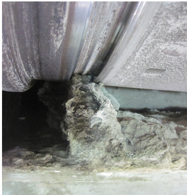
Figure 2-2. Nuisance Struvite Formation within Centrifuges
