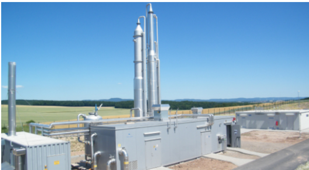
Figure 3-3. Wärtsilä's CA30LP amine system has a biogas treatment capacity of up to 550 scfm
