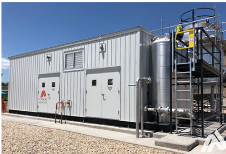
Figure 3-9. Unison membrane system treating 400 scfm of biogas at a WWTP
