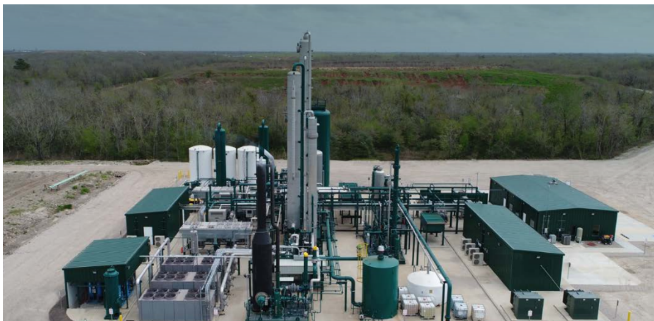
Figure 3-2. Morrow amine installation treating 12,000 scfm of biogas at a landfill
