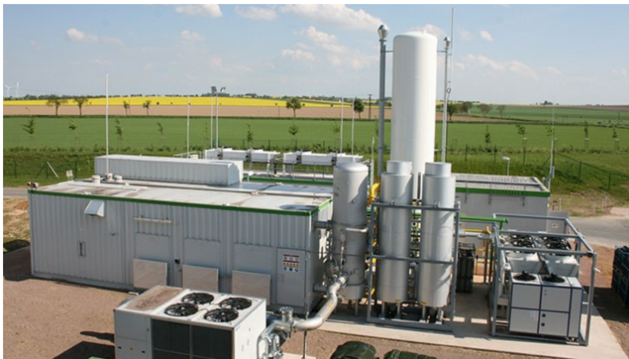
Figure 3-13. Carbotech PSA system treating 1,200 scfm of biogas
