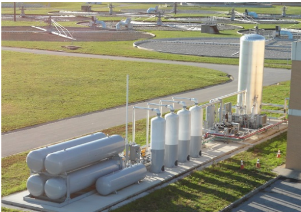
Figure 3-12. Guild PSA system treating 700 scfm of biogas at a WWTP
