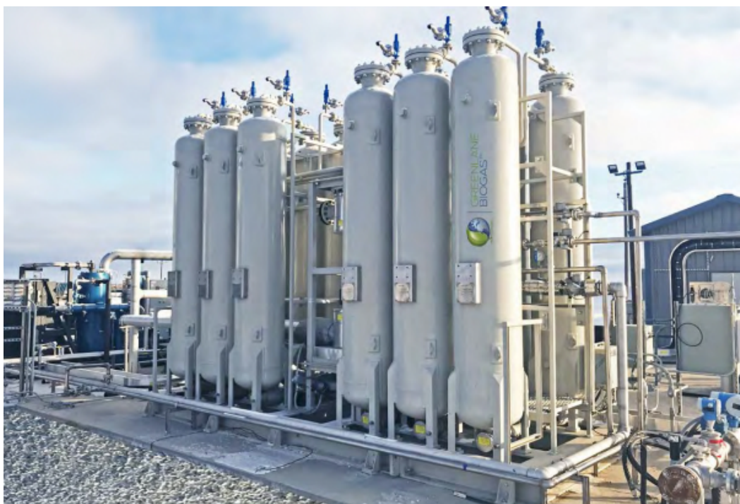
Figure 3-11. Greenlane PSA system treating 800 scfm of biogas at a dairy
