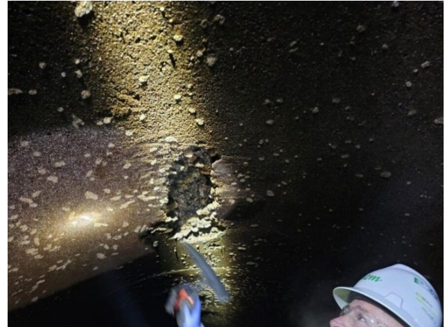
Deteriorated Concrete Tunnel Liner from 2015 on the left to 2024 on the right
