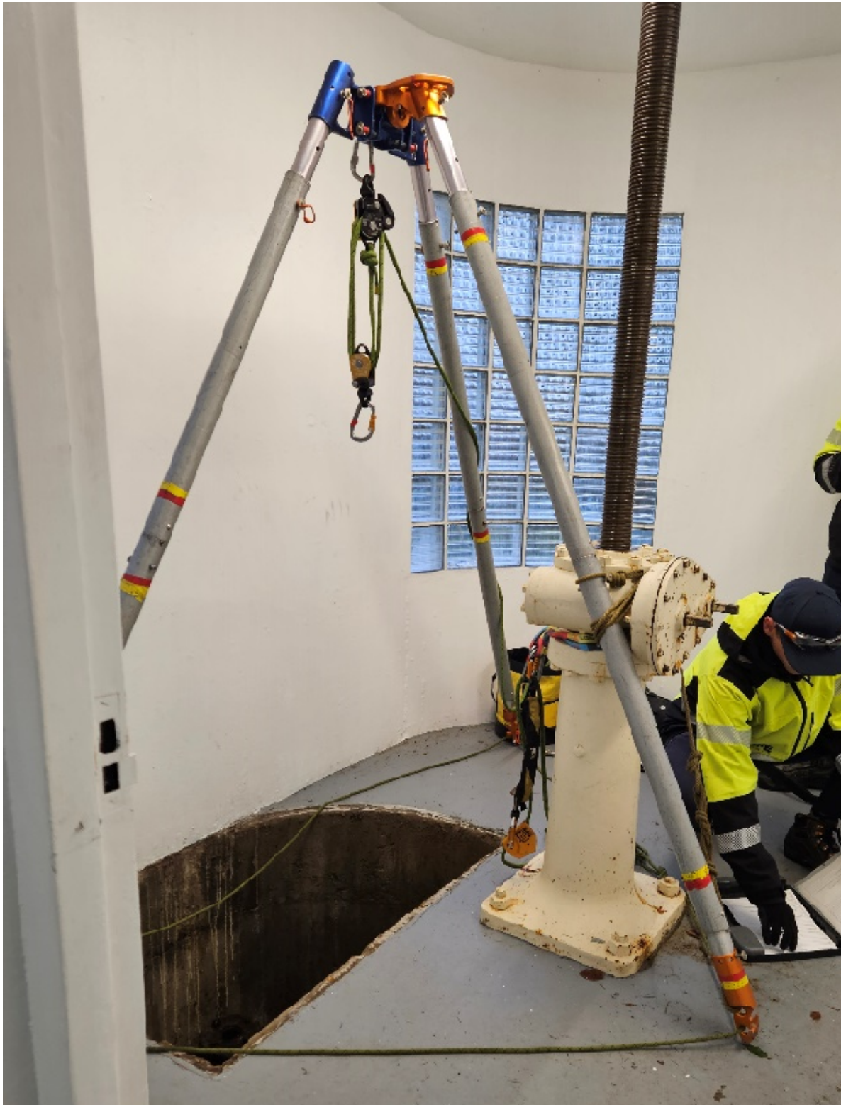
Figure 3: Confined Space Entry at Gatehouse
