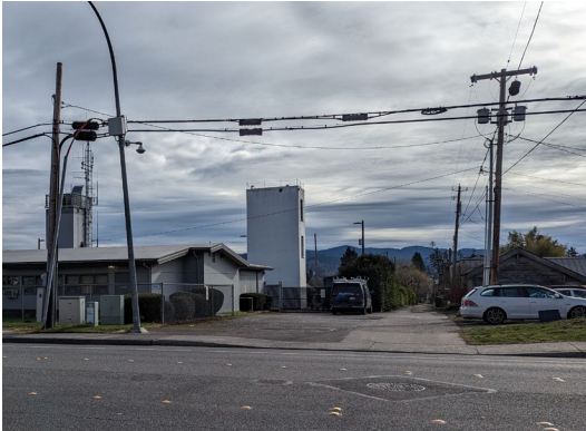
View of Alley - Looking North
