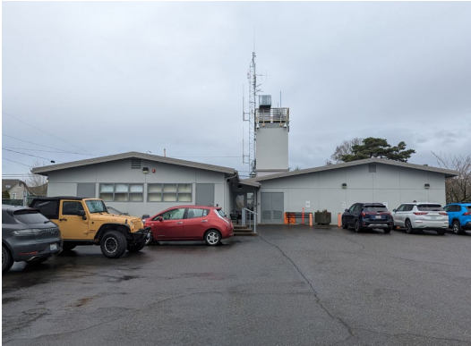
South Facade - Parking Lot
