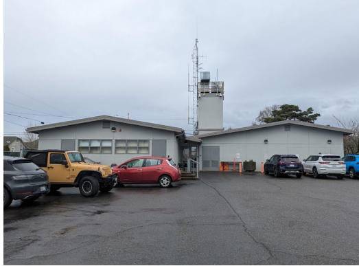
South Facade - Parking Lot
