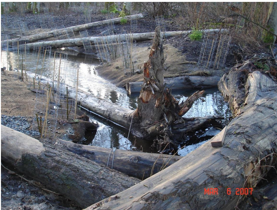
Figure 3-6 Photo showing recently constructed stream channel in Cemetery Creek, with newly planted conifers, willow stakes and deciduous shrubs; March 6, 2007.
