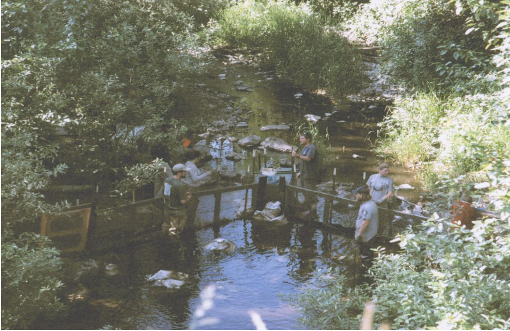
Figure 2. Picture taken during the dismantling of the smolt trap. Notice that water levels are below visquene on right side of weir. One of the pressure relief valves can be seen on the left side of the weir. The live box is at the center of the photo.
