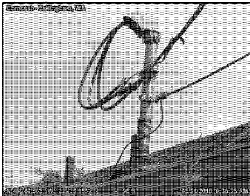
3235 Firwood Street, Cable drop attached to the power mast above the roof. Cables run over the roof of the building.
