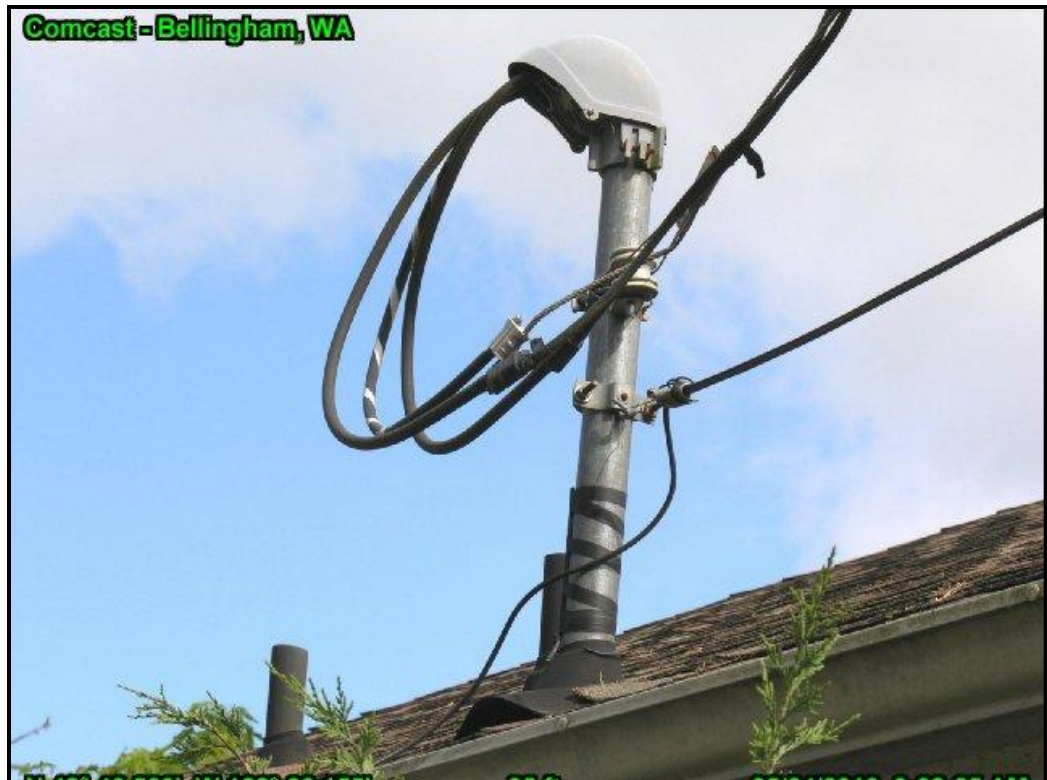
3235 Firwood Street. Cable drop attached to the power mast above the roof. Cables run over the roof of the building.
